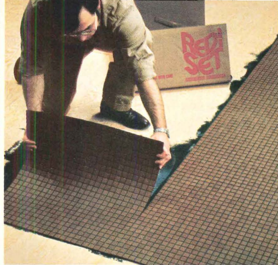
lay the pregrouted sheets,
