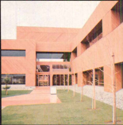
Redwood T&G lumber applied diagonally on office building complex
