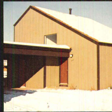
Ruf-Sawn 316 used as siding on low-income housing project in Colorado
