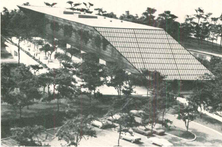
The North Carolina Blue Cross and Blue Shield Headquarters Building , by architects Odell Associates Inc., displays a new shape for reflective glass buildings—a 500-foot-long, 100-foot-wide rhomboid. Now being constructed on a 39-acre tract
