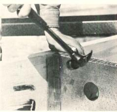
STEEL FLOOR JOISTS / End clips nailed to standard band board hold joists in position. Stairway and fireplace openings are formed by heading the joists. Hanger brackets support headers and tail joists. Decking is added and secured by self-tapping screws. ■ Armco Steel Corp., Middletown, Ohio.
