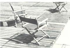
**REDWOOD PATIO DECK** / Preassembled units simplify installation and permit rearrangement or complete relocation with minimum effort.
