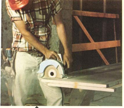
Panel ends are trimmed on-site with conventional equipment. Gold Bond Metaledge Corewall comes in panels 2 inches thick, 2 feet wide and up to 16 feet long.
