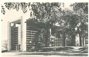
Power Center for the Performing Arts by Kevin Roche John Dinkeloo and Associates provides the University of Michigan with a \$3.5-million, 1,420-seat theater in a structure of reflective glass and steel reinforced concrete. The stage is convertible from proscenium to thrust by moving a lift for the orchestra platform which can stop at four levels. Jo Mielziner was the lighting and stage co-designer.
