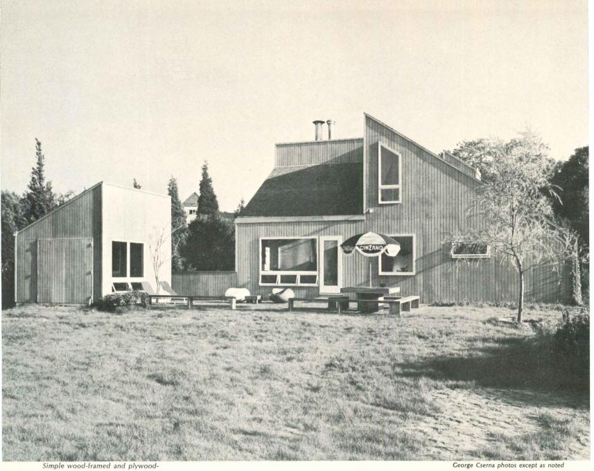
Simple wood-framed and plywood-clad volumes provide a lively interplay of form and shadow throughout the day. A trellis (below) at the entrance and the guesthouse provide varying degrees of spatial enclosure outdoors. Indoors (opposite page) a well-placed window bathes the living room wall with afternoon sun. The hexagonal brick pavers are used both indoors and on the terrace.
