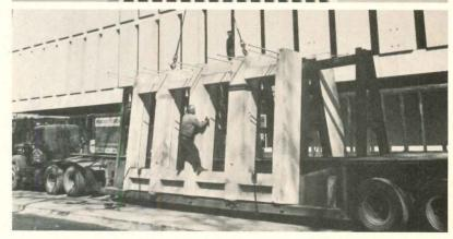
Precast load bearing units are 19'-11%" wide x 11' high. Average weight 12 tons. Spandrels are covered with black glass to accent vertical mullions.
