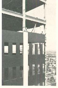
Martin Tower, Bethlehem Steel Corporation's new office tower in Bethlehem, has a unique curtain wall of panels fabricated from 3/16-in.thick steel plate. Pointed tabs projecting upward from the top of a panel are received by openings in the bottom of the panel above. The panels are locked in place and then they are welded at the sides to the building's columns and to angles along the beams.
