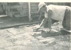
FLOOR SURFACING / Latex/cement material is said to withstand loads as great as 18,000 psi. Typical applications include indoor and outdoor loading docks and ramps, and storage areas. Permaflex Products Co., Philadelphia.
