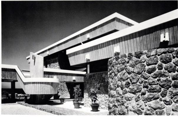
piers on 8-foot centers are important elements in containing the many views from these pavilions. The piers also relate the interior to the exterior concrete.
