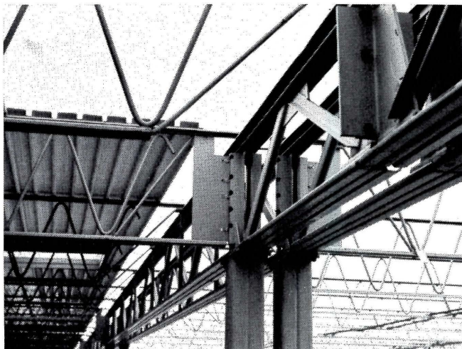
Macomber V-LOK connectors at the column lines . . .
