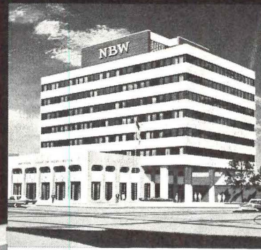
Laszlo Papp and Associates, architects ; R. C. Daly, construction consultant , Alexander-Jennings Construction Co., general contractor ; Consolidated Stone Setters, setting contractor .
