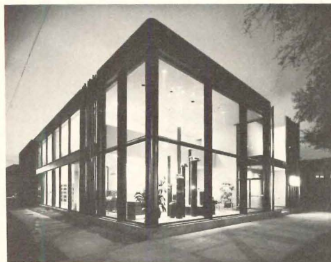
Olivetti Regional Office, New Orleans, The Olivetti Corporation of America Charles Colbert, Architect
