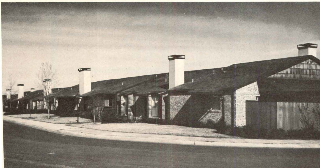
Brookgreen Town Houses, striking 230-unit development in Dallas. Imaginative planning includes efficiency town houses. Individually-controlled Lennox ducted electric heating and air conditioning; condensing units hidden from street. Architects: Ralph Kelman & Associates. Structural engineers: Chappell, Taylor & Mitchell. Owner/developer: I. C. Deal.
