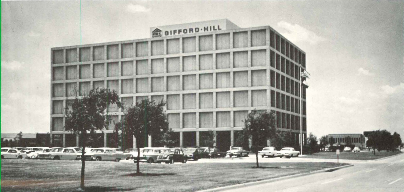
The new headquarters building for the Gifford-Hill Company in Dallas, Texas.
