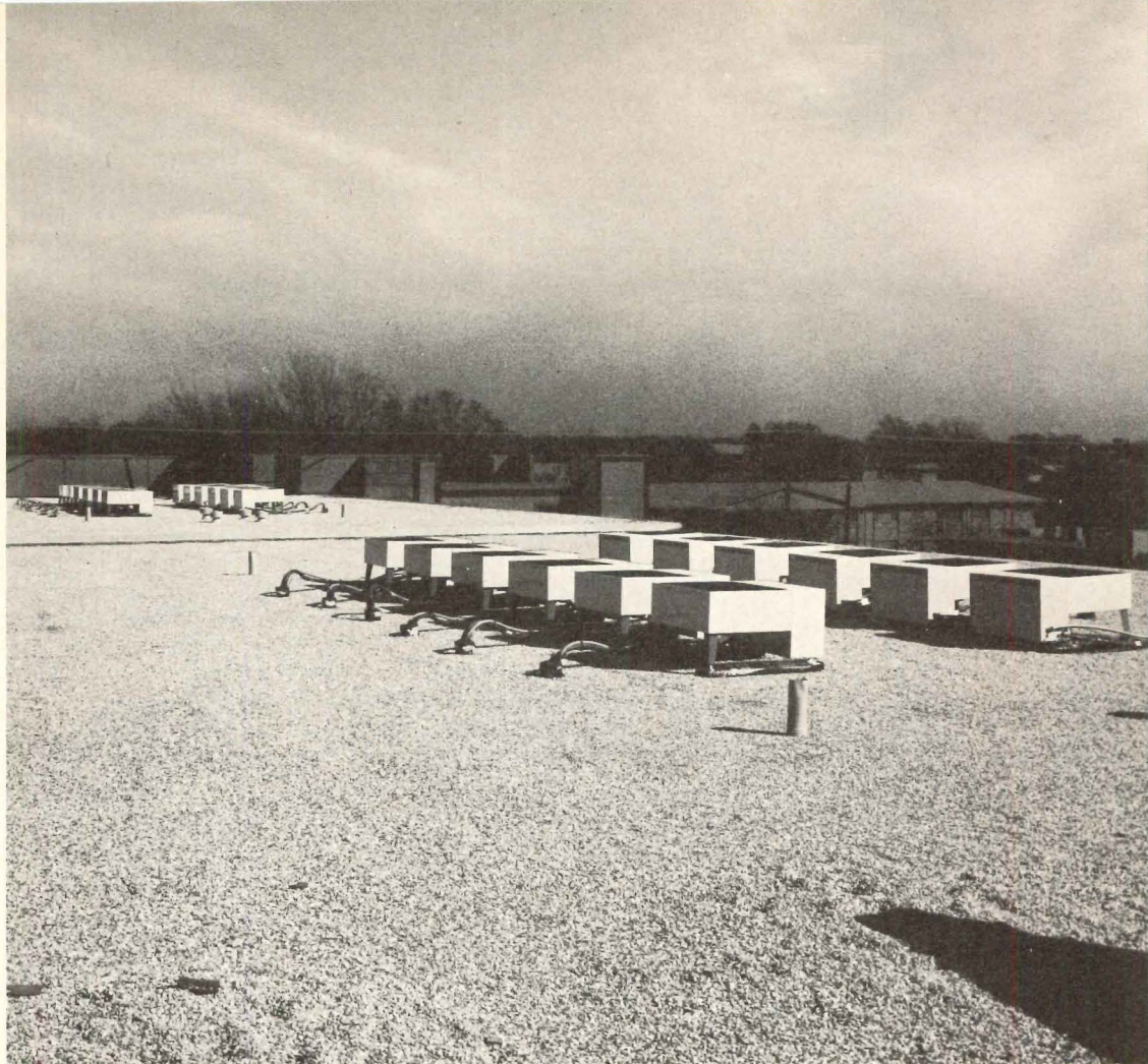
Mi Amigo Apartments, under construction in Dallas, is a complex of 149 apartments with individual ducted Lennox heating and air conditioning. New-design cooling units hide low on the rooftops. Architect: John Moss. Building Contractor: GTC Company. Heating/cooling contractor: Citywide Plumbing & Air Conditioning. Owners: George T. Connell and M. I. Harris, Jr.
