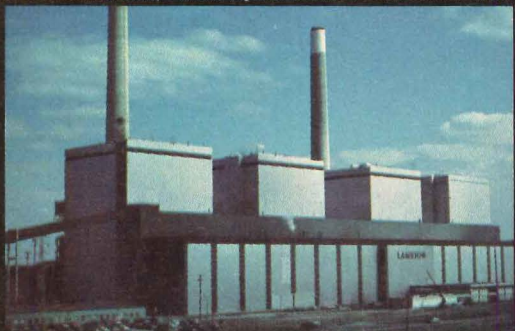
2. Lambton Station, Ontario Hydro Electric Power Commission.
