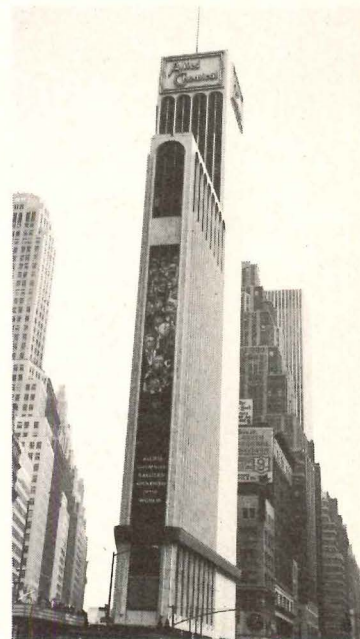
Allied Chemical Tower, N.Y.C. Architect: Haines Lundberg & Waehler, N.Y.C. Two-part LP® polysulfide based sealant in all joints of marble panels.
