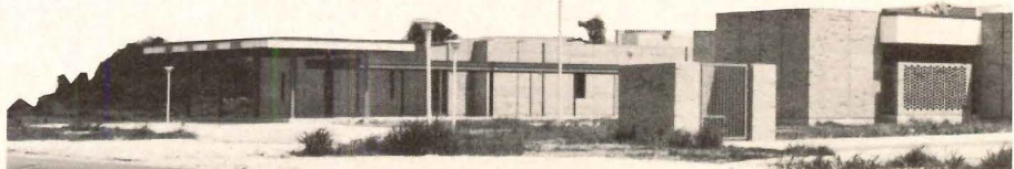
ARABI SCHOOL: Open, uncrowded spaces, excellent illumination, continuous-flow carpeting, soft coloring compensate for lack of window views in this Arabi, La., school where high humidity and high temperatures dictated a minimum of glass exposure. 315 tons of Lennox air conditioning serve 62,960 square feet of conditioned space. POWER SAVER™ unit cools free when outside temperatures drop below 57°F.
