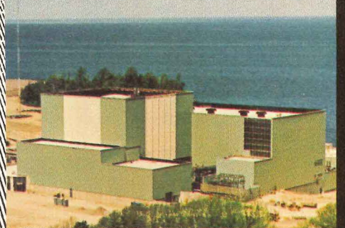
1. Ginna Nuclear Station, Rochester Gas & Electric Corp.
