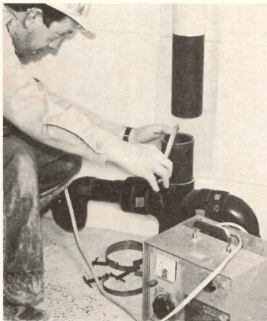
Polypropylene fittings and pipe for chemical wastes quickly joined with electrical fusion process.
