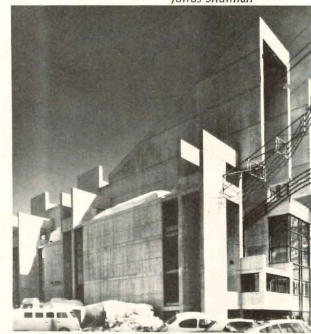
Squaw Valley Cable Car Terminal , Olympic Valley, California, Shepley Bulfinch Richardson and Abbott, architects, had to be a fireproof, earthquake-resistant building, supporting all the motive machinery for two 120-passenger cable cars, while serving as the anchor for the whole system, also providing ancillary facilities such as a ski rental shop.
