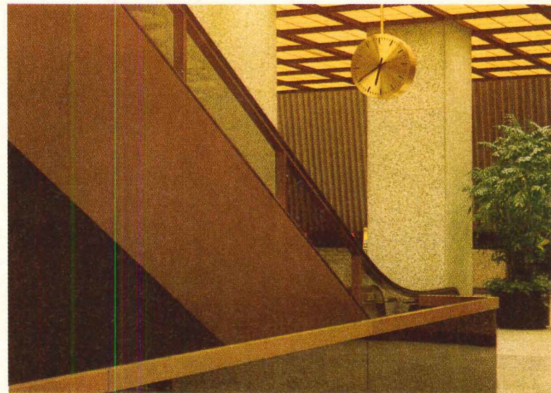
The beauty of bronze adds to the interior effect as escalator siding and railings.
