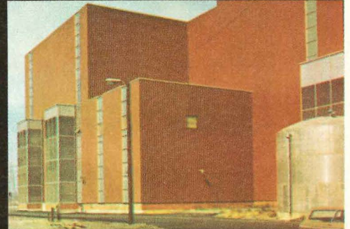
4. Trenton Channel Plant, Detroit Edison.
