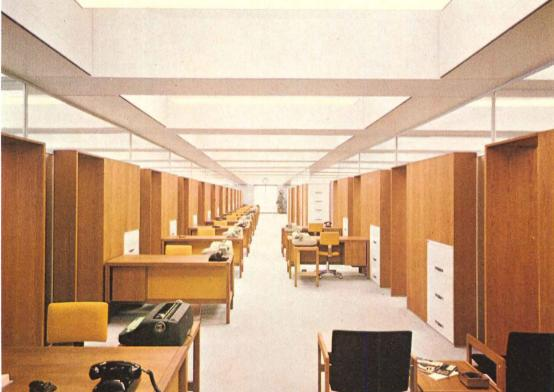
The ceiling grid—structural beams crossed by air-conditioning ducts-is left exposed, economically providing unusual spaciousness for office areas: under beams, height is 8 feet 8 inches; between beams, 11 feet. In the coffer thus produced, 7 feet square, a single light fixture is sus-
