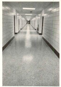
POURED SEAMLESS FLOORS / Florock is essentially a three step process in which the base coat is poured out, rolled and scattered with chips while still wet. When dry, a liquid polymeric glaze is applied, sanded and reapplied several times. Florock floors are said to be easy to clean, weather resistant, not subject to yellowing, durable and able to maintain their luster for years. ■ Crawford Laboratories, Chicago.
