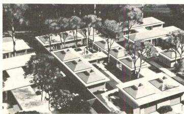
Republic Steel Corporation. Steel is the principal structural material in this system; it is formed into components to provide a variety of detached, single-family residences for low- and moderate-income occupancy. The system permits relatively high density single-family arrangements with privacy, and so is probably more appropriate for an in-city site than "detached residence" makes it sound. Kitchen-bathroom units are preassembled and set in place.
