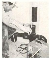
Polypropylene fittings and pipe for chemical wastes quickly joined with electrical fusion process.
