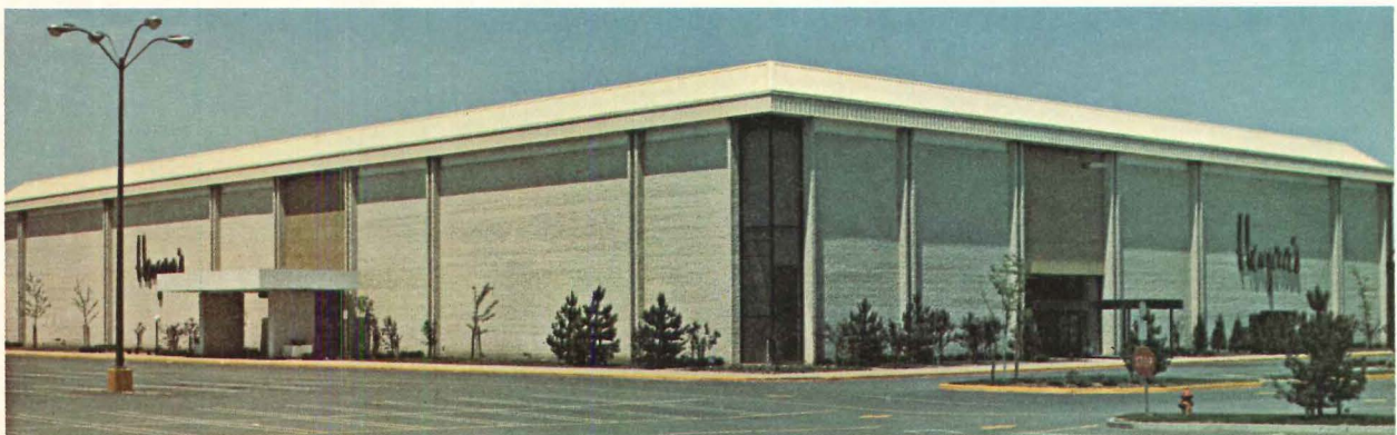
Hengerer's Department Store, Seneca Mall, West Seneca, New York. Architect: Herbert E. Johnson Associates, Washington, D.C.
