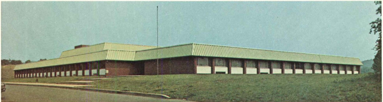
Quigley High School, Baden, Pa./Architects: Joseph Bontempo & Associates, Rochester, Pa.
