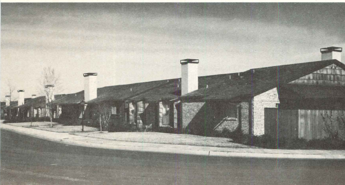
Brookgreen Town Houses, striking 230-unit development in Dallas. Imaginative planning includes efficiency town houses. Individually-controlled Lennox ducted electric heating and air conditioning; condensing units hidden from street. Architects: Ralph Kelman & Associates. Structural engineers: Chappell, Taylor & Mitchell. Owner/developer: I. C. Deal.
