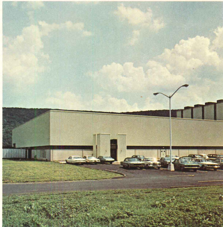
Westinghouse Electric Corporation, Industrial Plastics Division, Flexible Insulation Plant, Bedford, Pa. Archi- tects: Ingham Kaffka Marcu, Pittsburgh, Pa.
