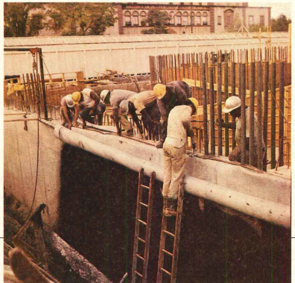
Workmen installing 20' x 90' Butyl sheets to form watertight sack before foundation was poured. Butyl sheeting material manufactured by Carlisle Corporation, Carlisle, Pennsylvania.
