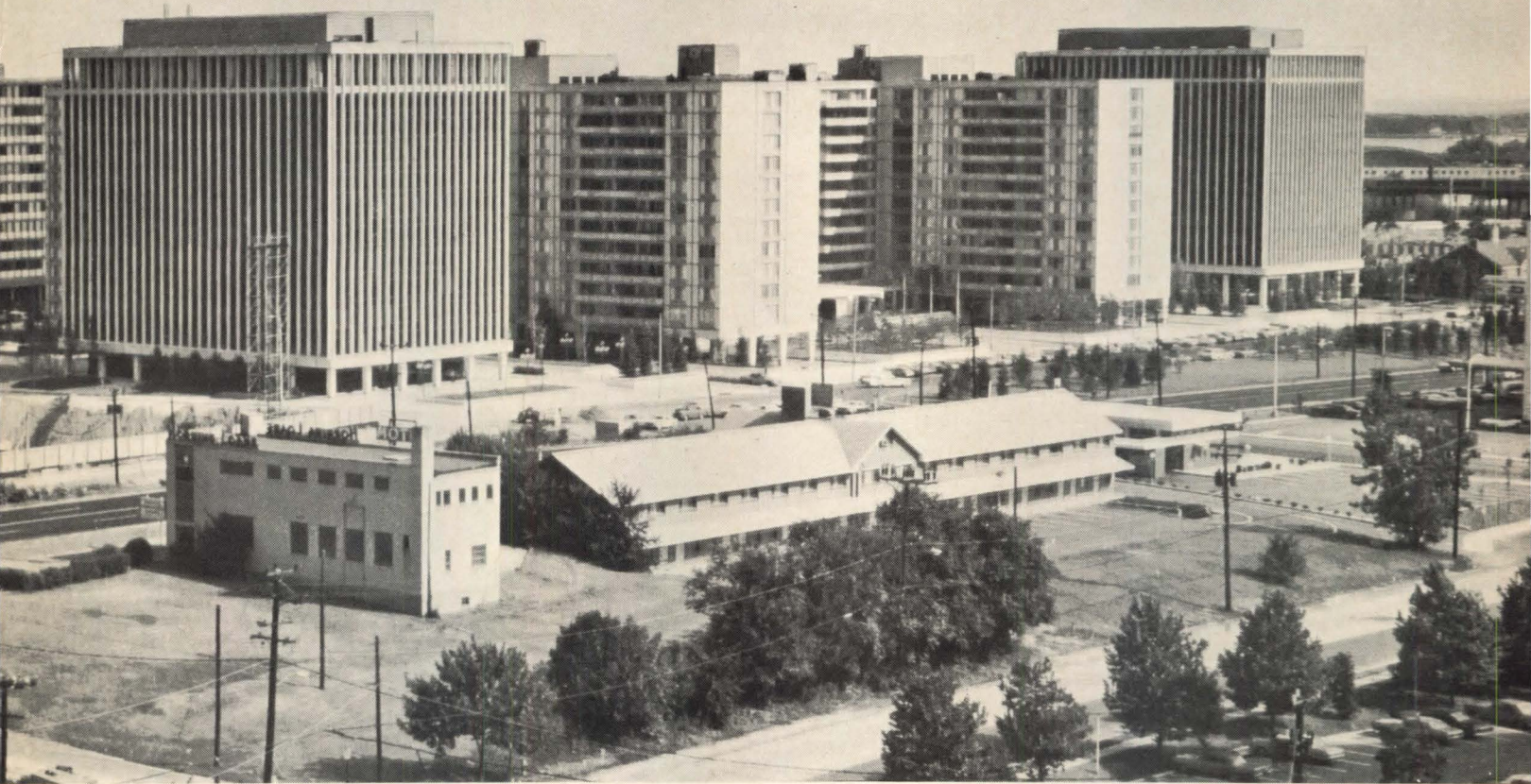
Ceco Steelform Service for 790,000 sq ft of monolithic concrete joist construction 12,700 tons of Ceco-fabricated Reinforcing Steel 480,000 sq ft of Cecocolor Anodized Aluminum Windows and Curtainwalls
