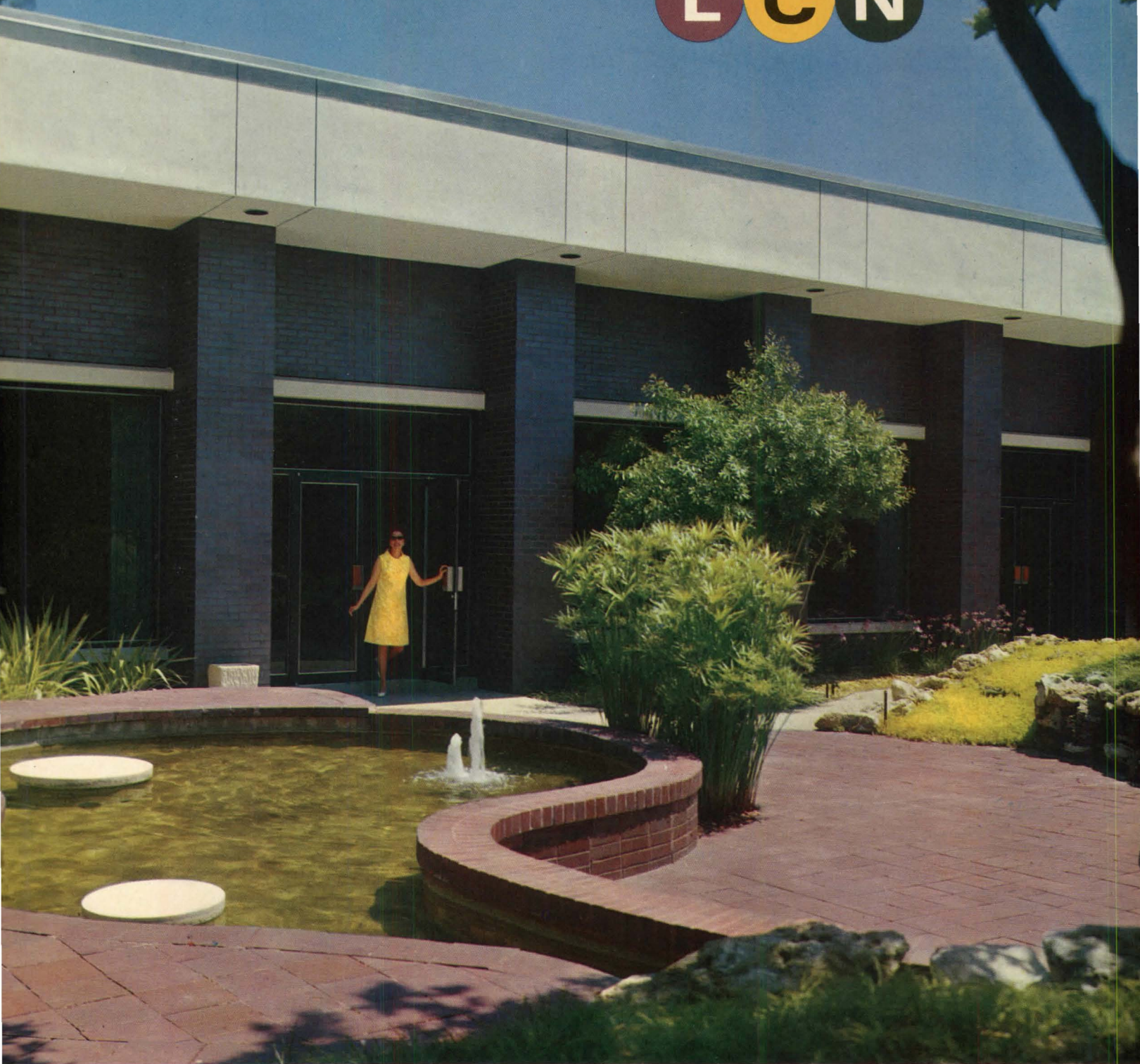
Overseas Operating Center, American Telephone and Telegraph Company—Long Lines Department, Jacksonville, Florida. Reynolds, Smith and Hills, Architects—Engineers—Planners; Jacksonville.
