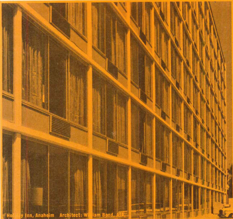
Holiday Inn, Anaheim Architect: William Bond, AIA
