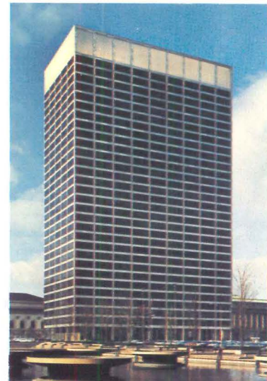
26-story Main Place (left), Buffalo, tops a 3-story shopping mall. Both were framed in steel to provide large, column-free areas and to simplify changing of floor layouts. Tower architect: Harrison and Abramovitz.
