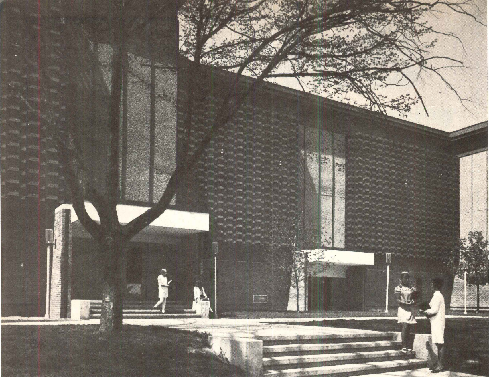
ARCHITECT: WARREN HOLMES CO., LANSING, MICH. ERECTOR FOR SCREEN: PAYNE-ROSSO COMPANY
