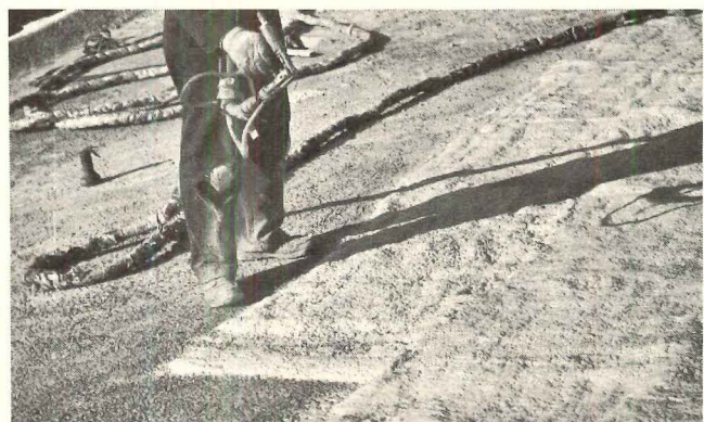
The 1" layer of urethane was applied to 98,000 sq ft by 3-man crew. Foam was later sealant-coated for added durability.
