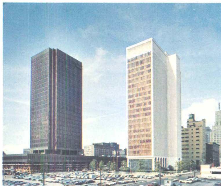
26-story Main Place (left), Buffalo, tops a 3-story shopping mall. Both were framed in steel to provide large, column-free areas and to simplify changing of floor layouts. Tower architect: Harrison and Abramovitz.
