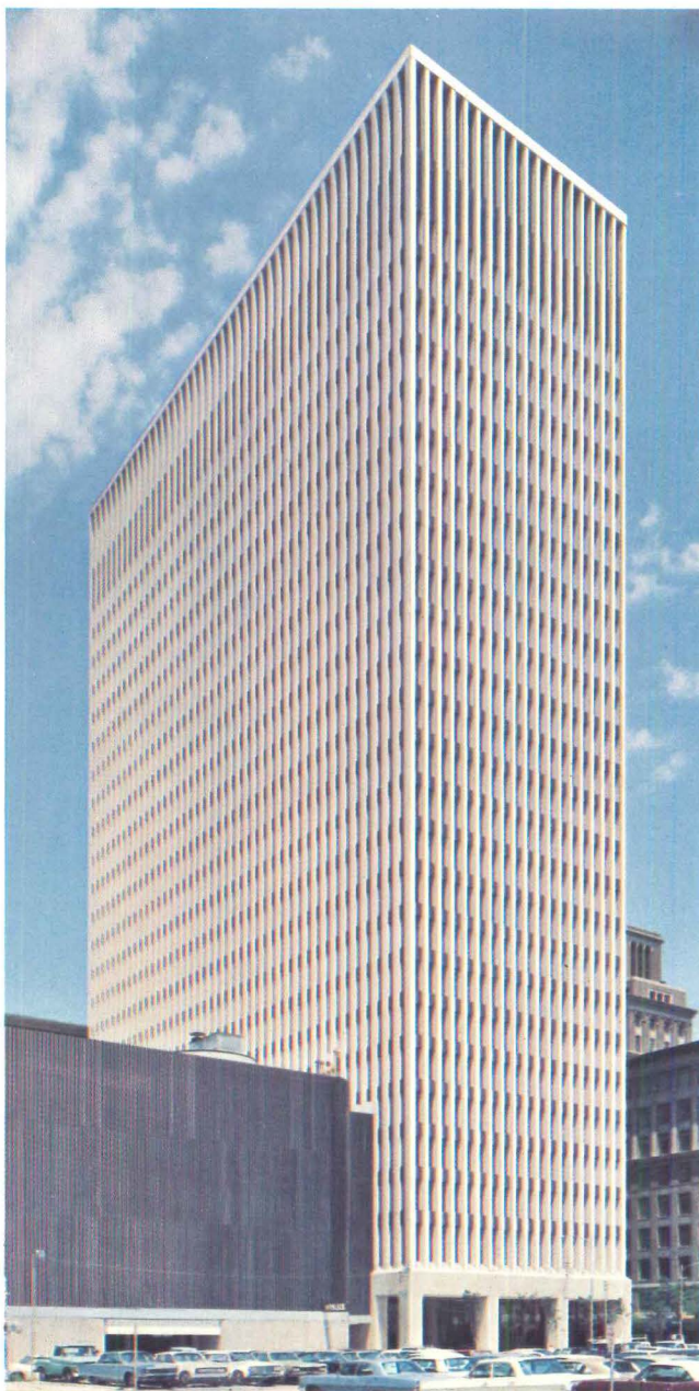
28-story Houston Natural Gas Building. ASTM A572 steel used in columns and beams for economy. Architect: Lloyd Morgan and Jones, A.I.A.
