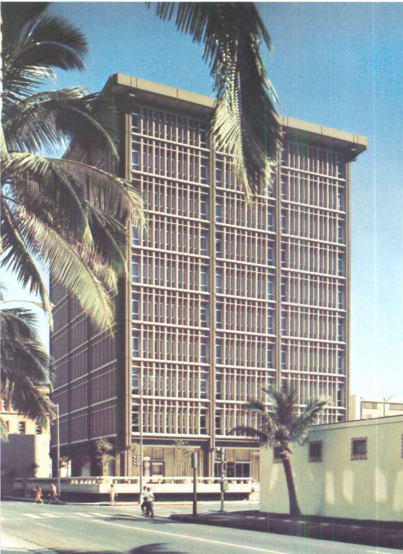
10-story City Bank of Honolulu, an AIA honor award winner, features a fully electrified floor system and 30 x 30 ft bays. Architect: Takashi Anbe, A.I.A., Walter Tagawa, A.I.A.
