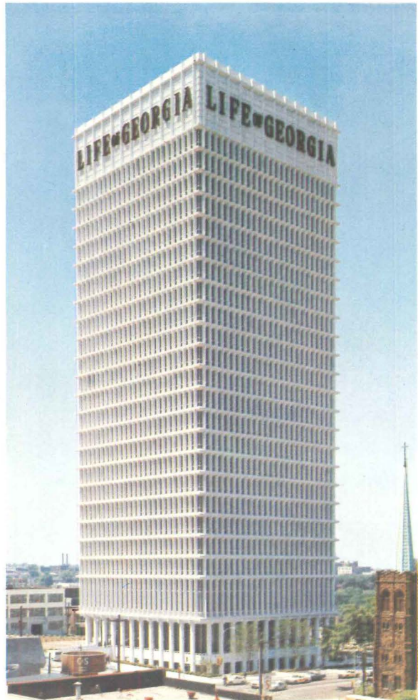
29-story Life of Georgia Tower, Atlanta. Steel permitted slender columns for architectural effect and was ideally suited to the cellular steel flooring system which gives tenants complete office-area flexibility. Architect: Bodin & Lamberson.
