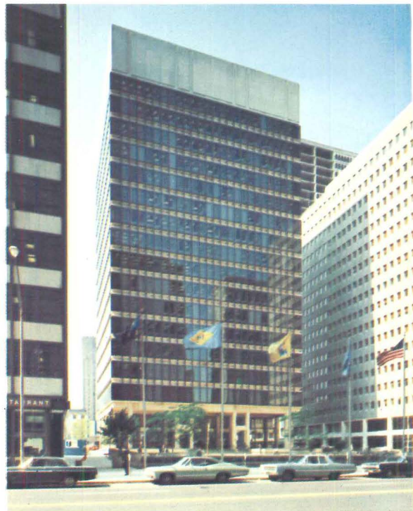
21-story IBM Building, Philadelphia (15 glass-enclosed office floors). Offset service core (not shown) serves as the backbone and steel framing serves as the rib cage to provide unusual openness and flexibility of space. Corrugated steel underfloors contain built-in channels for telephone and electrical wires. Architect: Vincent G. Kling, FAIA.
