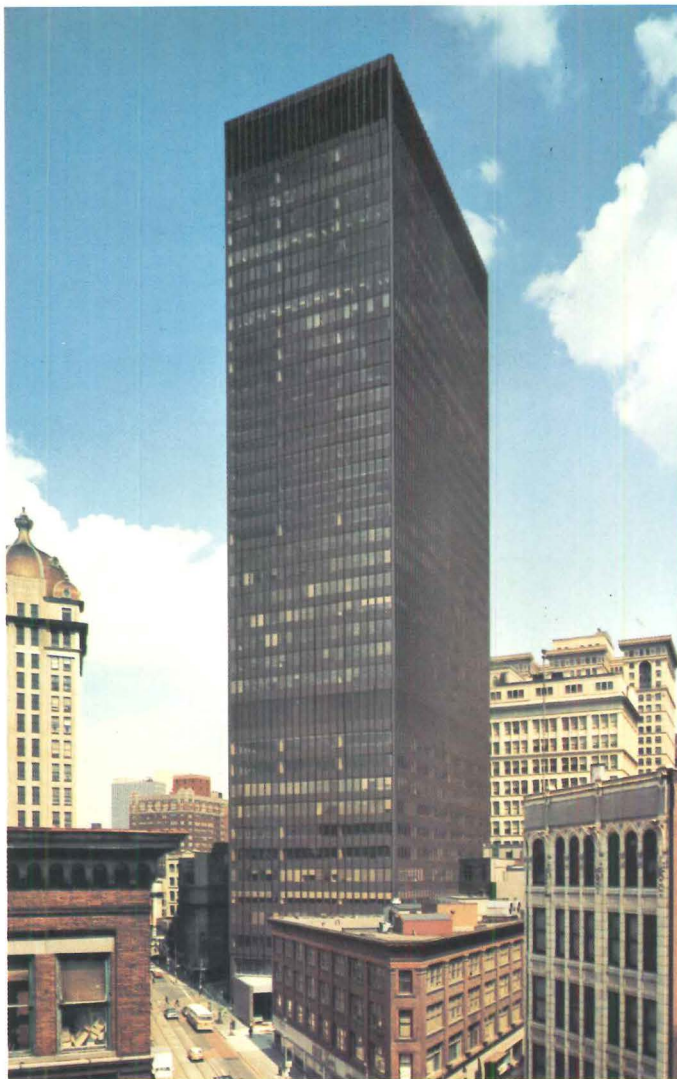
39-story One Oliver Plaza, Pittsburgh. Steel framing chosen for speed and economy of construction; big, column-free areas; cellular steel floor decking. Steel framing also made it easy to make changes to answer tenant needs. Architect: William Lescaze and Associates.
