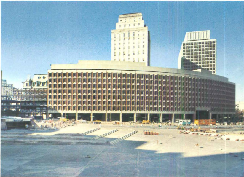
8-story One Center Plaza, Boston, which is being built in three phases (three 300-ft sections). Steel framing was chosen for the ease with which it can be expanded laterally, and for the interior flexibility it provides. Architect: Welton Becket, FAIA.
