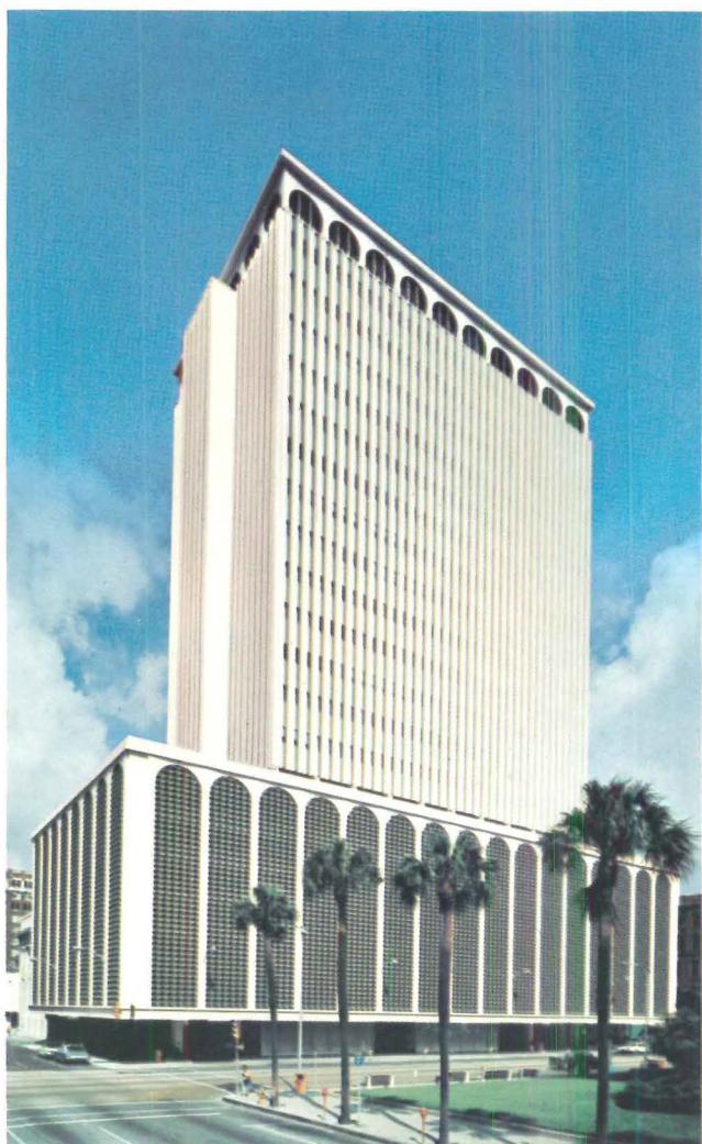
22-story Exchange National Bank Building, Tampa. Redesign in ASTM A572 steel (grades 50 and 55) saved $45,000. Floor framing in office tower section is designed compositely with the slab. Architect: Harry A. MacEwen, A.I.A.
