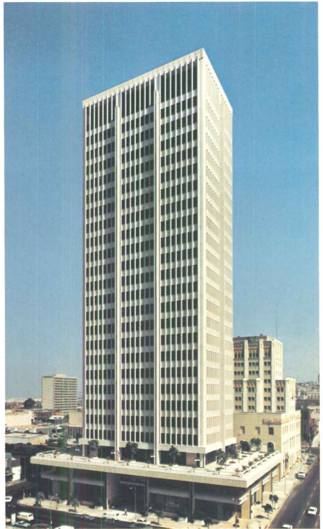
25-story First National Bank Building, San Diego. Steel framing helped to meet extremely fast schedule of just 21 months from architect's conception to start of occupancy. Architect: Tucker, Sadler & Bennett.
