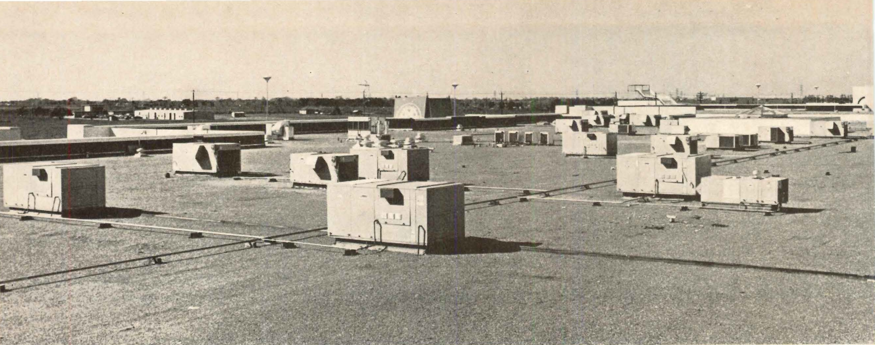
Typical installation of Lennox single-zone combination gas heating/electric cooling system for large, undivided spaces. Also available for oil or electric heating. Installs on rooftop—or at grade level.
