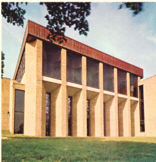
The functional and highly decorative band which terminates Agudath Sholom Synagogue (left and above) in Stamford, Conn., is an excellent example of a typical copper fascia. Architects: Davis, Brody & Associates.
