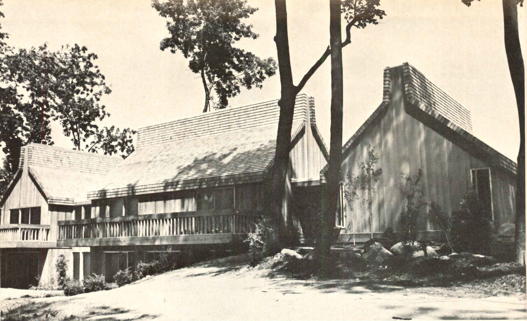
Architect: Delnoce Whitney Goubert Builder: Frank H. Taylor and Son, Inc.
