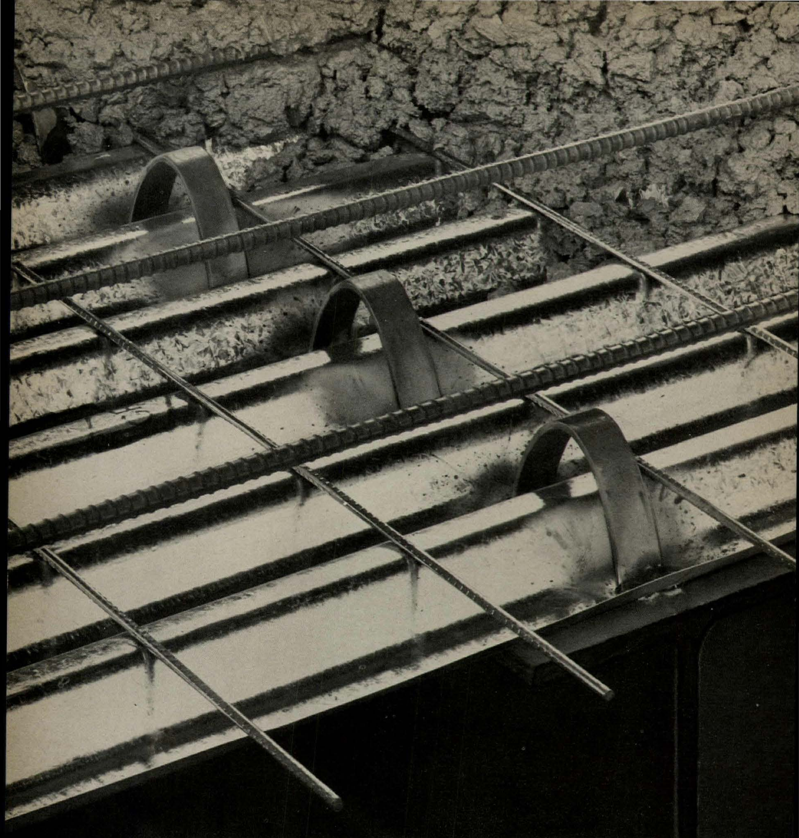
Typical Placing Patterns on Girder
