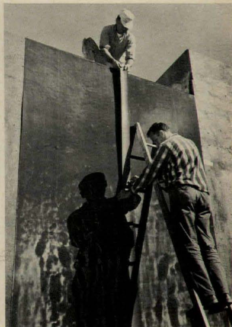
Floor, walls and roof of underground computer center are sheathed with neoprene membrane. Walls are primed, and a neoprene bonding agent is used.
