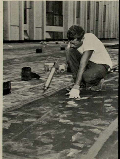
Approximately one acre of neoprene sheet covers this plaza and waterproofs the library building below. Neoprene putty reinforces seams.
