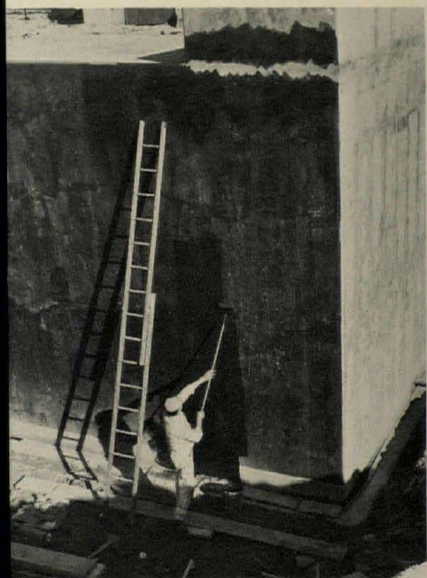
Floor, walls and roof of underground computer center are sheathed with neoprene membrane. Walls are primed, and a neoprene bonding agent is used.
