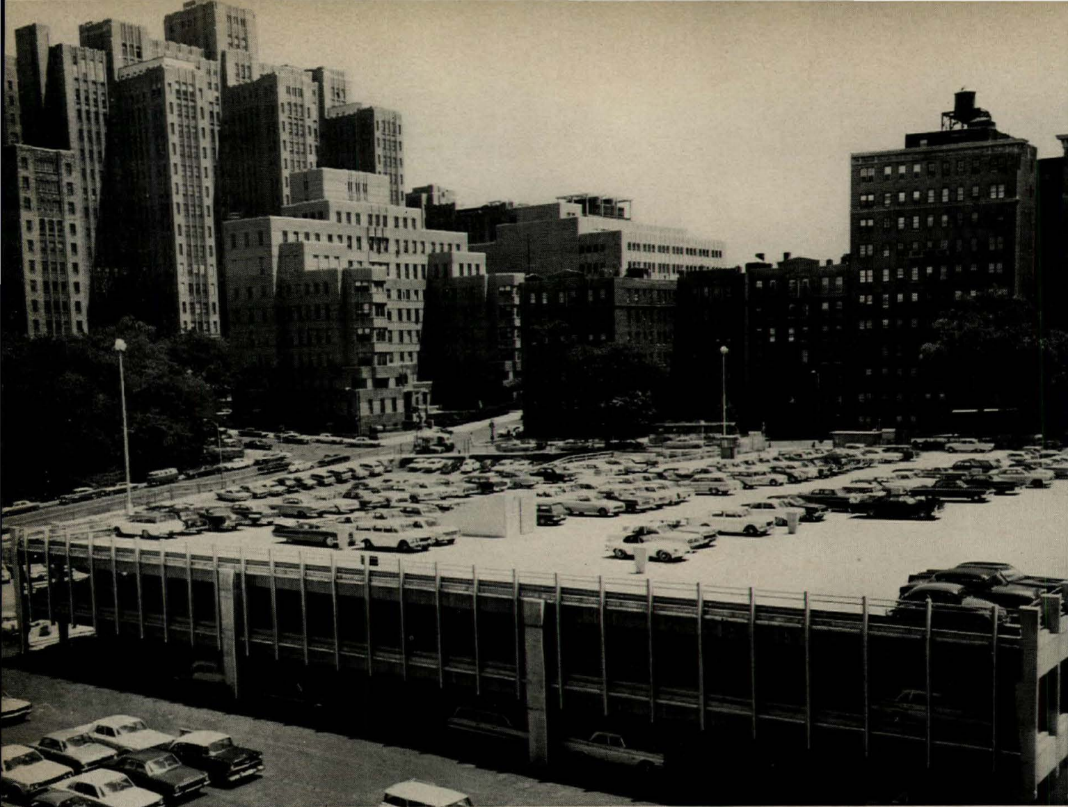
COLUMBIA PRESBYTERIAN MEDICAL CENTER GARAGE, New York, N.Y. Architects and Engineers: EDWARDS & KELCOY, Newark, N.J. General Contractor: W. J. BARNEY CORPORATION, New York, N. Y. Precast, Prestressed Concrete: BLAKESLEE PRESTRESS, New Haven, Conn.
