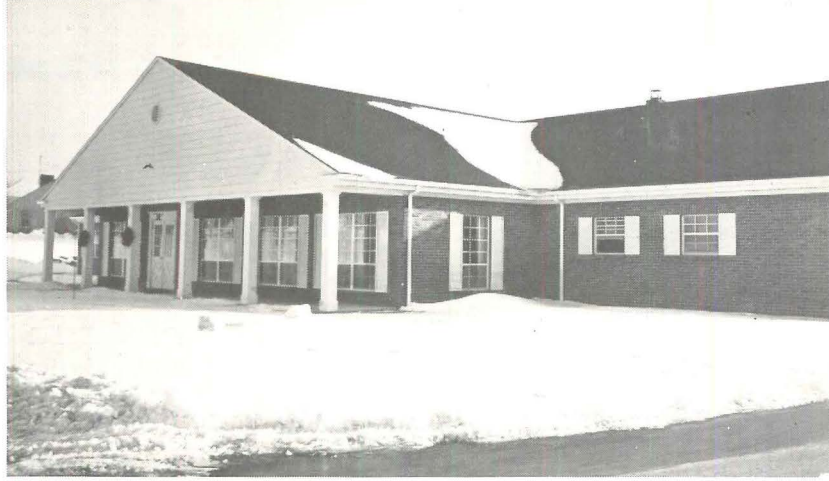
$20,000 SAVING: 19,000 sq. ft. Den-Mar Nursing Home, Rockport, Mass. Architect: Di Meo Associates, Stoneham, Mass. Engineer: Joseph Sestito & Associates, Malden, Mass. Contractor: Feldman Construction Co., Rockport, Mass.
