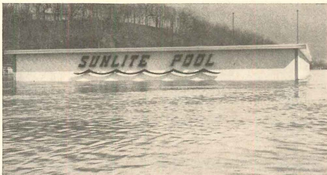
After the flood water receded, the canopy was completely unharmed! Canopy was prefabricated of Ruberoid T/NA 200 and stressed-skin plywood by Batavia Plywood Fabricators, Inc., Batavia, Ohio. The Sunlite Pool is part of Coney Island Amusement Park in Cincinnati.
