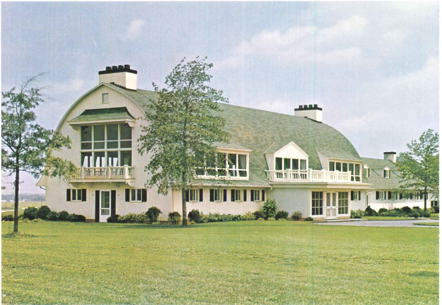
Hominy Hills Country Club, Colts Neck, New Jersey. Architect: Derick B. Kipp, A.I.A., Montclair, N.J. Builder: Charles Hagerman, Colts Neck, N.J.
