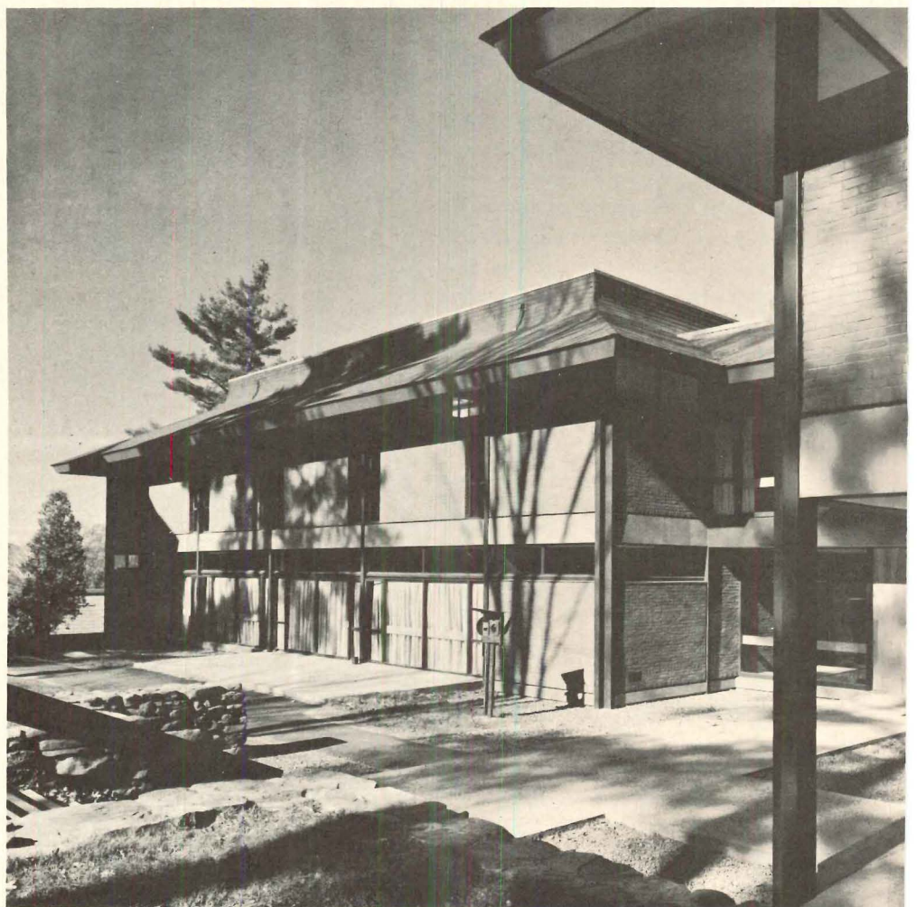
A small "link" building connects the library and classroom blocks. The main floor of the link consists of
