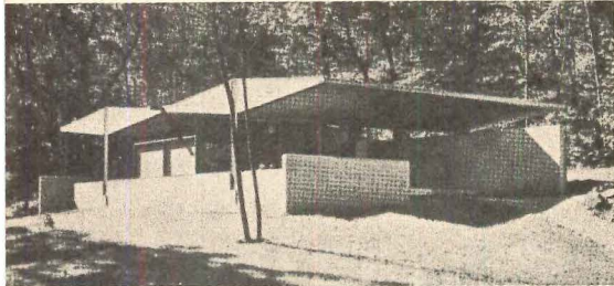
1956: Franzen's own house places airplane-roofed glass pavilion on light podium. Julius Shulman
