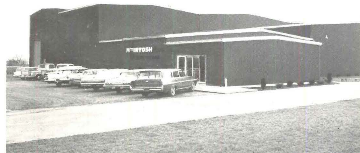
$7,000 SAVING: 9,400 sq. ft. McIntosh Stamping Corp. plant, Berne, Ind. Designer/Builder: David Poor Construction Co., Warsaw, Ind. Engineer: Berne Electric Co., Berne, Ind.
