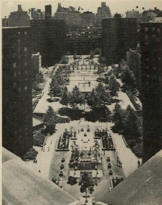
Award for Merit in Landscape Architecture and Urban Design: Carver Houses Plaza, New York City Architect: Pomerance & Breines Landscape Architect: M. Paul Friedberg General Contractor: Cuzzi Bros. & Singer
