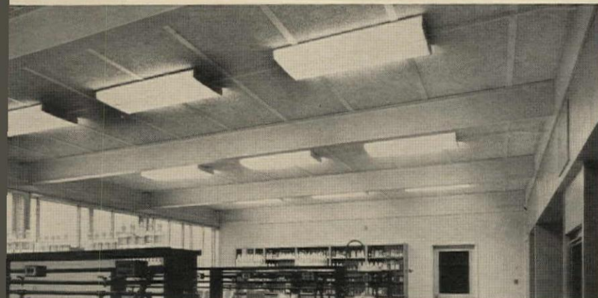
Tectum eliminated need for additional acoustical treatment in most classroom areas. Drop ceilings were needed only in corridors and on lower floors under concrete slab.
