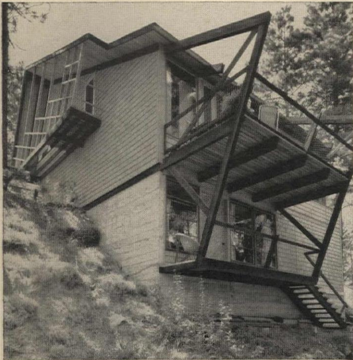
The imaginative use of cantilevered beams supports the double-deck sun deck. The open styling never obstructs the panoramic view of the countryside. The wide windows help to bring the view indoors as well.
