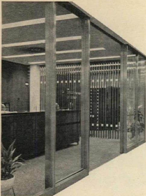
National Bank of Detroit, by architects Albert Kahn and Associates. Stainless steel vault screens, sliding doors and partitions.
