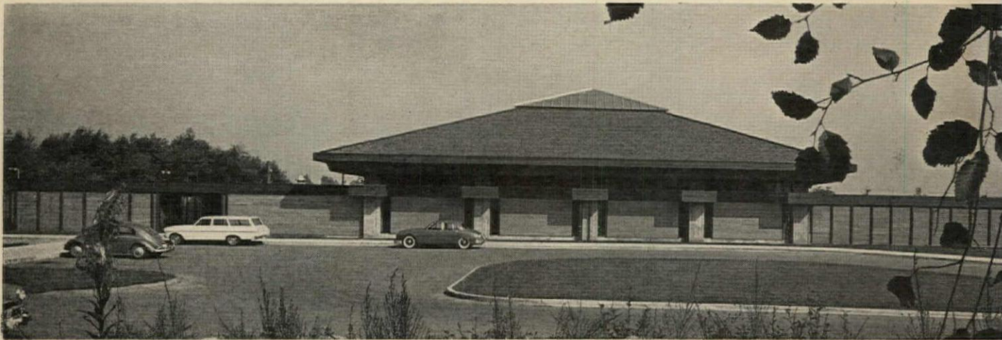
C. J. Brown Memorial Pool, Burnaby, British Columbia Architectural and Structural: McCarter, Nairne & Partners Pool equipment: McCarter, Nairne & Partners Heating and Consulting: D. W. Thomson & Company Ltd., Consulting Mechanical Engineers Electrical: R. Lennox Mackenzie, Consulting Electrical Engineer General Contractor: Biely Construction Company Ltd. Owner: Corporation of the District of Burnaby
