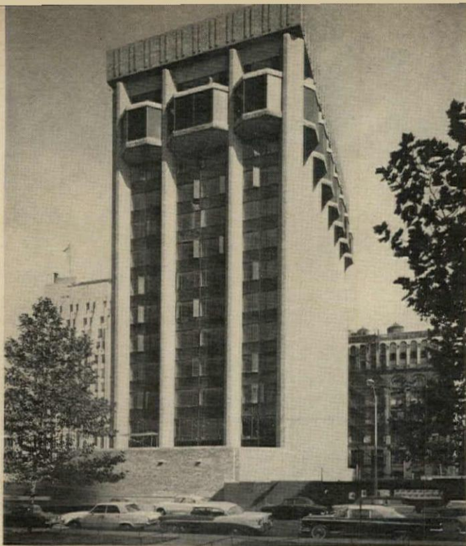
First Honor Award for Excellence in Civic Architecture and Urban Design: Warren Weaver Hall, Courant Institute of Mathematical Sciences, New York University Architect: Warner Burns Toan Lunde Structural Engineer: Severud-Perrone-Fischer-Sturn-Conlin-Bandel Mechanical Engineer: Meyer, Strong and Jones General Contractor: Wigton-Abbott Corporation
