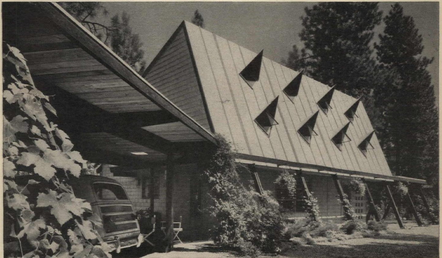
The unusual diamond-shaped window styling of this home near Tacoma, Washington, features a peaked sunshade over each dormer window for a distinctive studio appearance. Architects: Warren Cummings Heylman & Associates.
