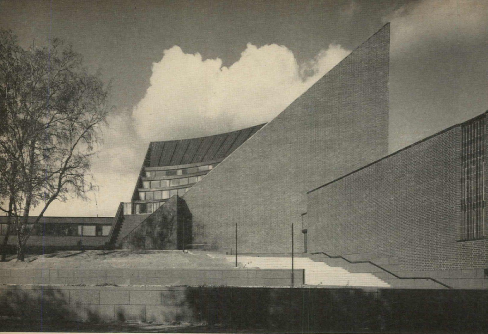
Stair to terrace and outdoor amphitheater
