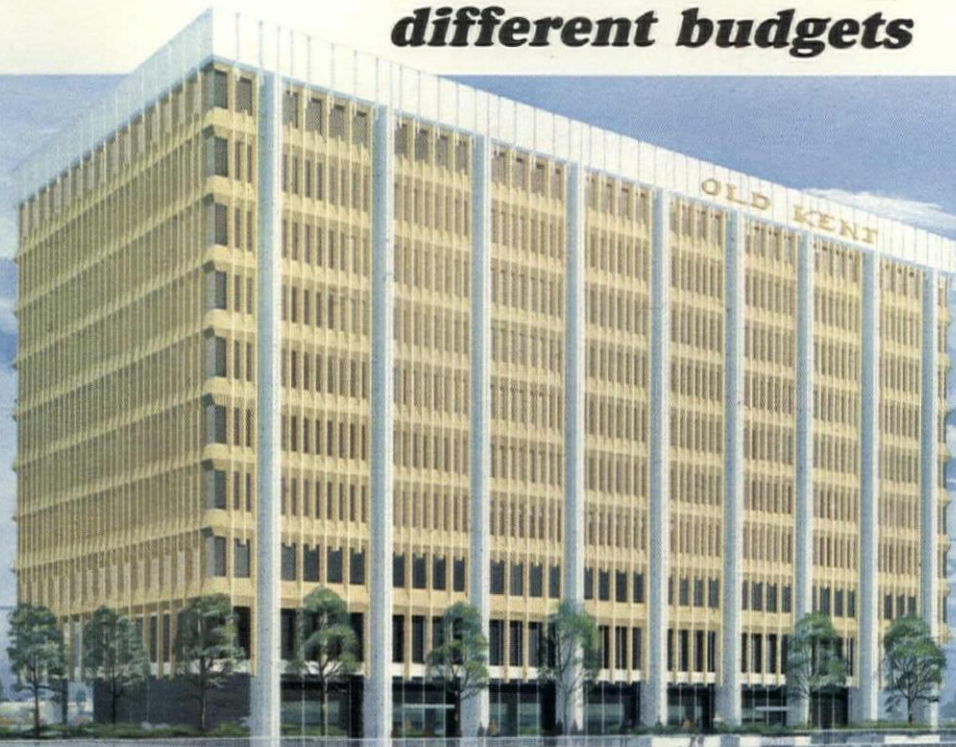
Old Kent Bank and Trust Company, Grand Rapids, Mich. Architects and Engineers: Daverman Associates General Contractor: Owen-Ames-Kimball Co.
