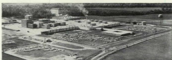
This all-glass roofing system was topped with Fiberglas Perma Ply and Perma Cap roofing felts.
