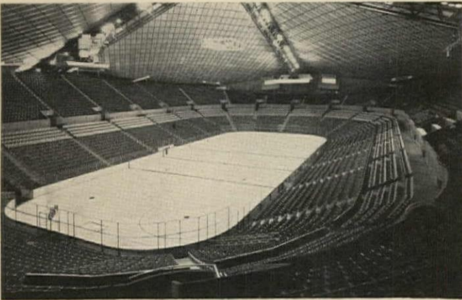
Category: Best Design in Low-rise Commercial, Industrial or Institutional Construction—Seattle Center Coliseum Architect: Paul Thiry, F.A.I.A. Structural engineer: Peter H. Hostmark Mechanical engineers: James B. Notkin and Associates Electrical engineers: Beverly A. Travis & Associates General contractor: Howard S. Wright Construction Company
