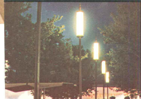
Specially designed decorative pylon lighting creates atmosphere and mood on exterior walks and concourses. Used as supplementary lighting to give soft illumination.
