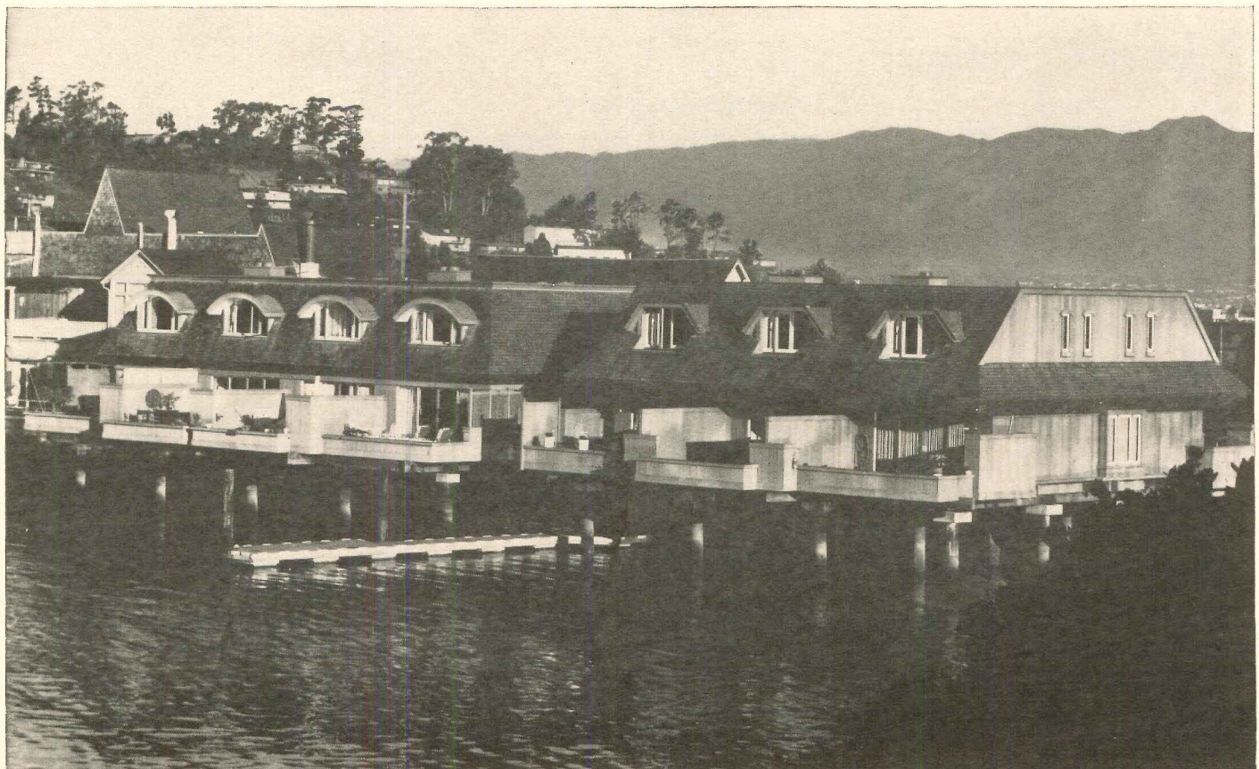
Wood, first wedded to water by early shipbuilders, goes modern with today's homebuilders. Pole construction of the Cove Apartments in Belvedere, California, withstands wind and weather. Owner: Belvedere Land Company. Architect: Charles Warren Callister,
