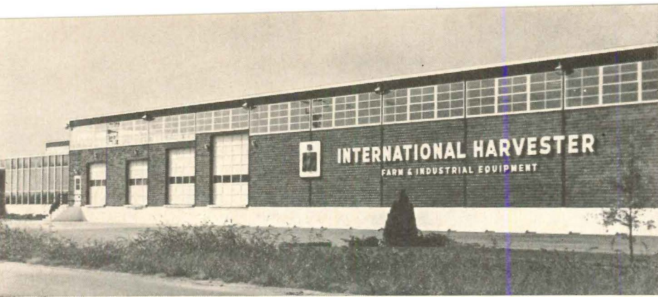
EFFICIENT PLANT, KANSAS —International Harvester, Wichita. Architect: Campbell Engineering Company. Prime Contractor: A. W. Soderberg Construction Company. Masonry Contractor: Kenneth D. King. Masonry Cement: United Cement Products Company. Concrete: Dolese Bros. Company.
