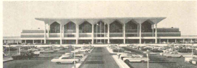
Memphis Metropolitan Airport, Memphis, Tennessee Architects: Mann & Harrover Structural Engineers: S. S. Kenworthy & Associates Mechanical and Electrical Engineers: Allen & Hoshall Graphic Design: Architectural Graphics Associates General Contractor: J. A. Jones Construction Company
