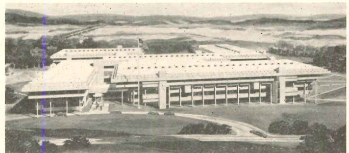
IBM Components Division, East Fishkil, N. Y., also by Rudolph and engineered by Kidde, another step toward functional expression (solid wall for mechanicals on second floor under cantilevered office space on top floor)
