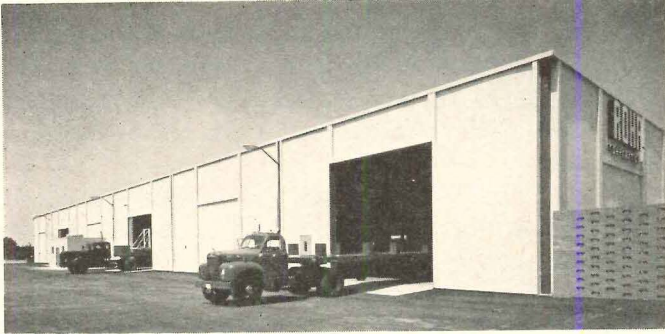
Back of the Rohr plant (page 174) shows removable concrete panels which can be re-assembled on future plant extension
