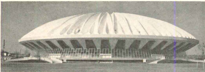
Assembly Hall, University of Illinois, Urbana, Illinois Architects: Harrison & Abramovitz Structural Engineers: Ammann & Whitney Mechanical Engineers: Syska & Hennessy Acoustical Engineers: Bolt, Beranek & Newman, Inc. Landscape Architects: Clarke & Rapuano Lighting: Abe H. Feder General Contractor: Felmley-Dickerson Company
