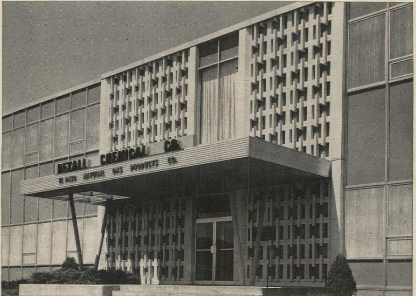
OFFICE & RESEARCH CENTER, REXALL CHEMICAL CO., Paramus, N. J. Finne-Lyman-Finne, architects. Weny Bros. & Storms Co., builder. To create this distinctive perforated facade, the architects designed their own grilles in architectural terra cotta. Eight-inch thick through-wall units with plastic insert were formed by two 4" thick white grilles.
