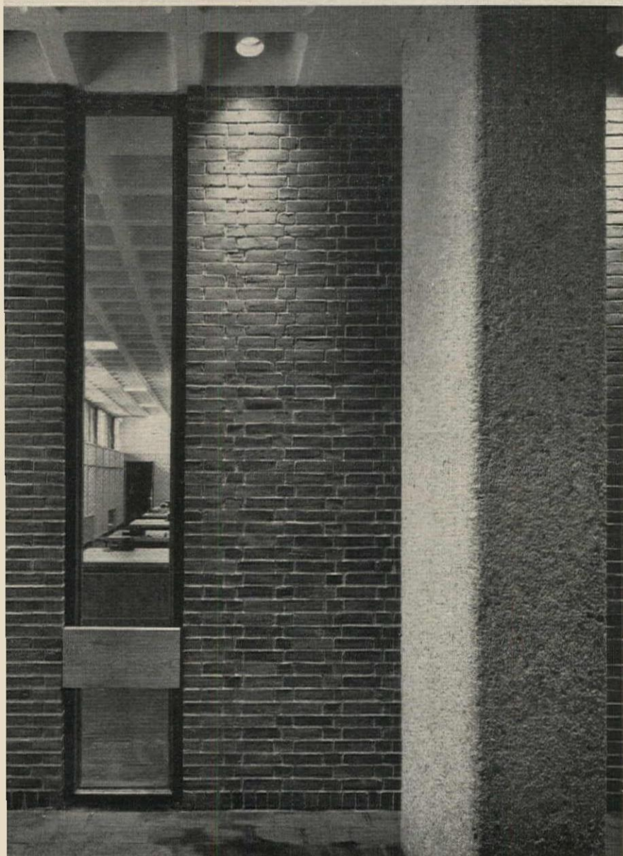
Exterior detail ( left ) shows careful coordination of wall and window with waffle module
