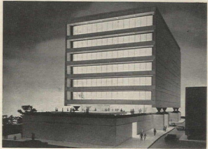
American Republic Insurance Company Building, Des Moines; Skidmore, Owings & Merrill, architects; Paul Weidlinger and Associates, structural engineers. "We were intrigued with the concept of the precast, prestressed floor structure which spans between the long walls, a matter of 99 feet, and were equally intrigued with the floating effect of the superstructure over a powerful statement of walls at street level . . ."
