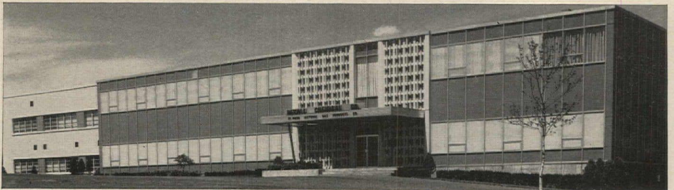
OFFICE & RESEARCH CENTER, REXALL CHEMICAL CO., Paramus, N. J. Finne-Lyman-Finne, architects. Weny Bros. & Storms Co., builder. To create this distinctive perforated facade, the architects designed their own grilles in architectural terra cotta. Eight-inch thick through-wall units with plastic insert were formed by two 4" thick white grilles.
