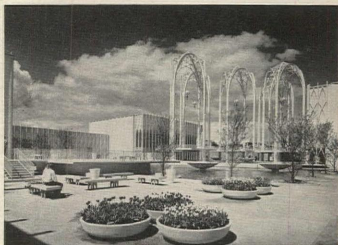
U.S. Science Pavilion , 1962 World's Fair, Seattle; Minoru Yamasaki and Associates, and Naramore, Bain, Brady & Johnson, associated architects; Worthington, Skilling, Helle & Jackson, structural engineers. ". . . a very exciting form, climaxed by the free standing interlocking arches . . . a virtuoso performance showing what can be done with concrete—what previously would have been done with wood or steel"
