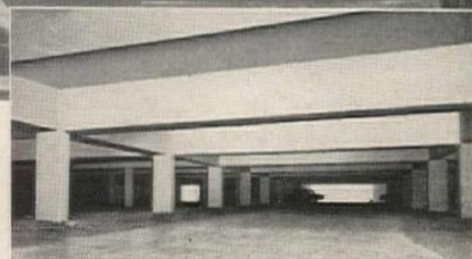
Post-tensioned beams used in underground parking garage.
