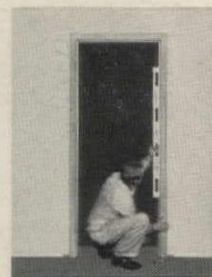
4. Square and anchor in place as shown
