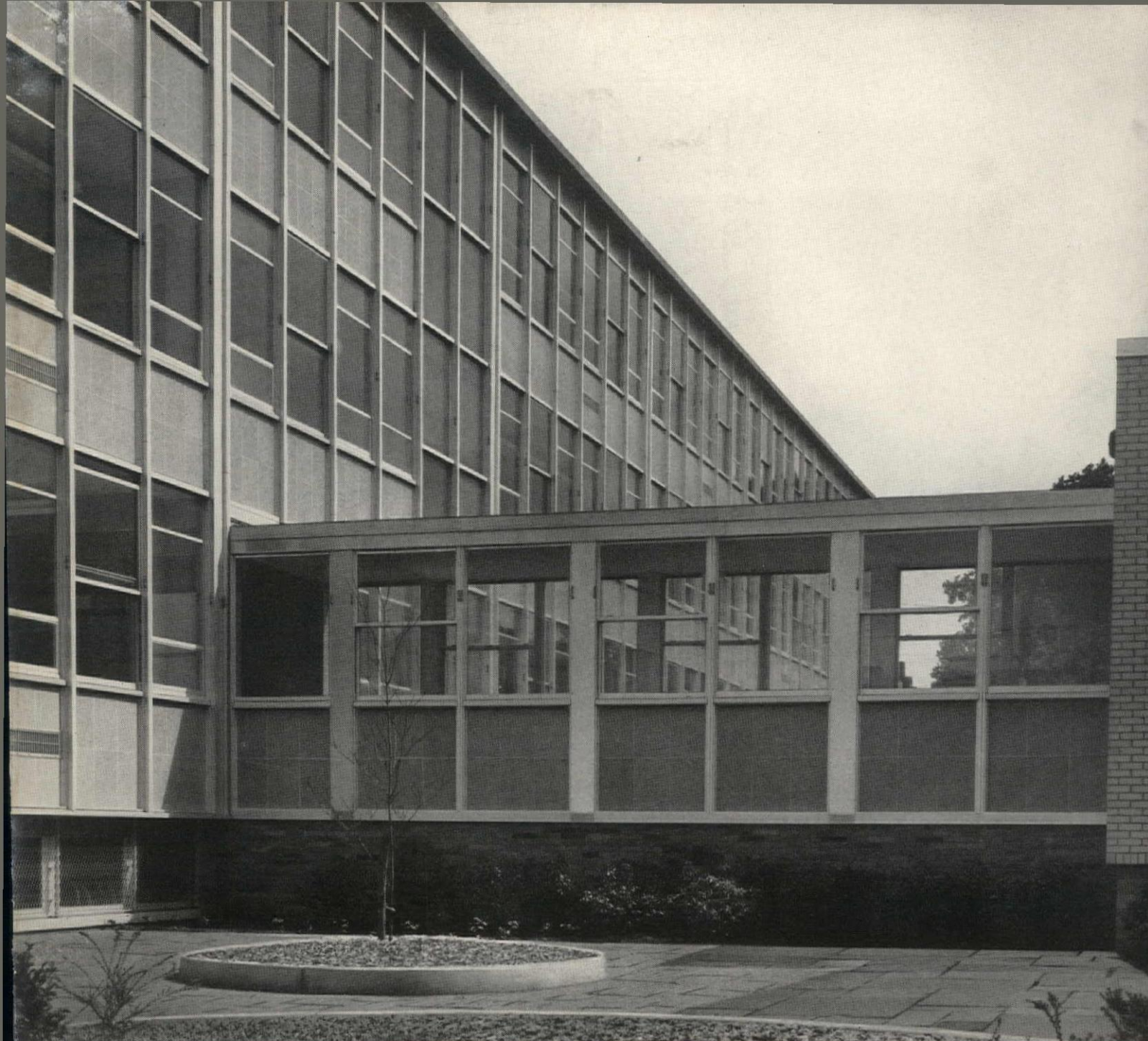
P.S.40, Jersey City, N. J. Architect, Valdemar H. Paulsen, Jersey City. Panels, Panel Corp. of America, Danbury, Conn. Terra cotta, Federal Seaboard Terra Cotta Corp., N. Y.
