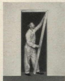
2. Slide on lock and hinge jambs
