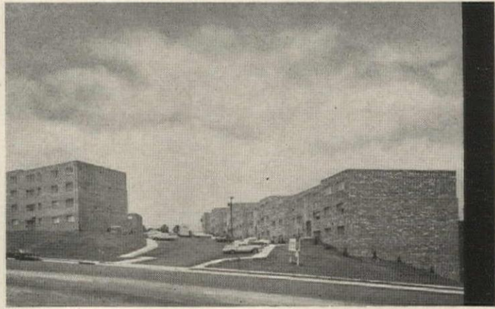
Typical installation—Bohn Apartment Units cool and heat these new apartments near Washington, D. C.
