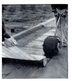
A new idea in built-up roofing consists of a 3-ft-wide mastic tape which is applied cold to flat or sloping surfaces. Under development at Koppers laboratories for more than four years, commercial production is expected later this year.
