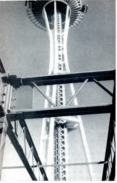
V-LOK framing interlocks without nuts, bolts or rivets. The Plaza Restaurant and Cocktail Lounge, one of the eight buildings with V-LOK framing, is shown below.
