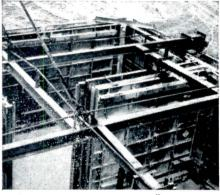
Lifting pads are welded to  $8^{\prime\prime}$  l-beams that tie assembly together. Tension rods strengthen unit and keep it square.
