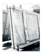
cast angle irons and stud bolts for attaching panels to bearing surfaces.
