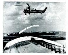
day. The roof, 150 ft above ground, has a 2- by 6-in. tongue and groove southern pine decking furnished by the Forest Products Div. of Olin Mathieson. Arches and purlins were pressure treated. Unit Structures, Inc., Pestigo, Wis.
