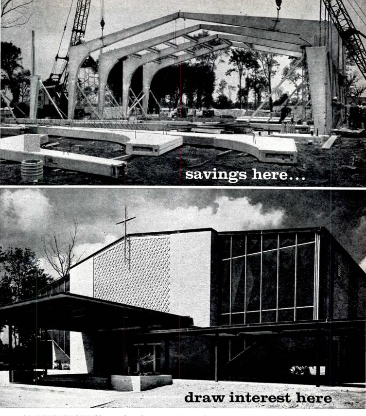
**CONSTRUCTION SAVINGS** are implicit where precast, prestressed concrete is employed—as in the framing for this auditorium of St. Andrew the Apostle Church in Algiers, La. Work goes fast, erection costs are low. The precaster further reduced costs by using 'Incor' 24-hour portland cement for the arches and roof joists. Incor's fast-curing properties permit speedier production, earlier release of forms. **OPERATIONAL SAVINGS** go on and on. By specifically choosing precast con-
