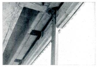
irons—here pictured—stud bolts near the bottom of the panels were secured to stud bolts in sill bottoms. Installation thus was fast, firm, and effective.
