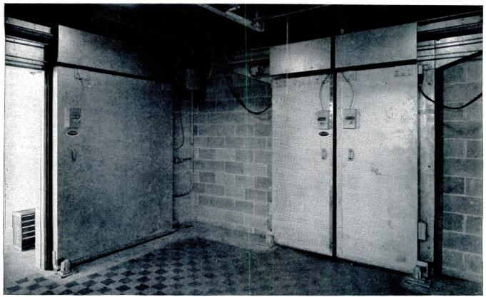
FAST OPENING AND CLOSING. Jamison Electroglide<sup>®</sup> Power Doors speed traffic to loading dock—single leaf cooler door, left, and bi-parting freezer door, right.
