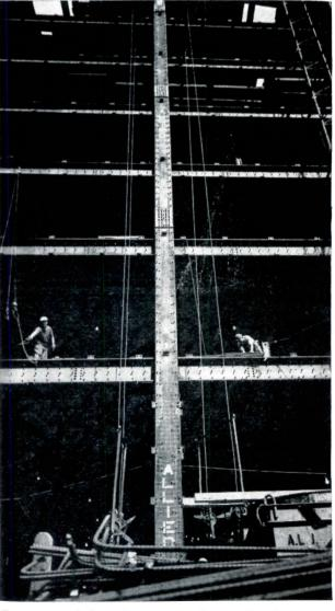
Covers are tied to the concrete fireproofing by means of stud anchors. Structural steel is A440 alloy. Stud anchors are welded to both plate and structural steel
