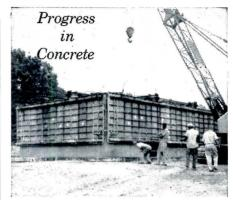
A complete form for concrete house being lifted by crane. The unit, of Symons Forms, has 5,000 square feet of surface.
