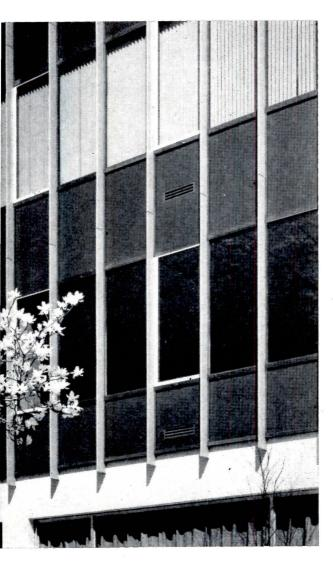
The structure of the 777 Summer Street building is steel frame with bar joist floor and roof construction. Floor and roof slabs are poured concrete on metal decking. Interior partitions are plastered concrete block, solid gypsum board or metal stud and gypsum board, painted or with vinyl wall covering. Flooring is terrazzo on the ground floor, asphalt tile on the stories above. Exposed grid, mineral acoustical tile is used throughout the building.
