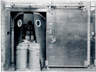
SAVES REFRIGERATION. Jamison Manual Horizontal Sliding Door in combination with self-closing Flexidor<sup>®</sup>.
