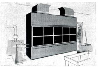
4. A 41E Weathermaker can provide heat in winter, too, by simply adding a special heating coil. Steam or hot water can be used from any source, or a small self-contained boiler can stand alongside the unit.
