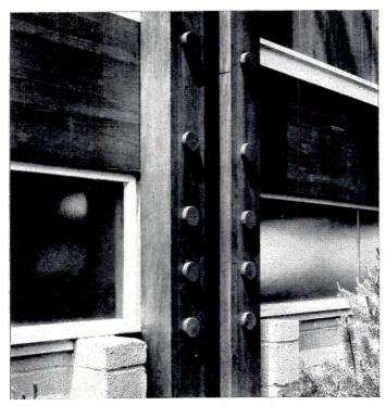
A close-up of the club's laminated posts shows off the inherent strength of wood in fist-sized pcg fastenings. This grass-high view also illustrates wood's compatibility with the barest forms of glass and concrete.
