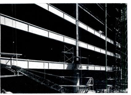
Welded carbon-steel plate covers have been applied over the spandrel beams. They will be protected from corrosion by paint
