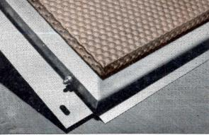
**CLOSE-UP** of one of the embossed panels showing brass strip braces to which panels are silver soldered.
