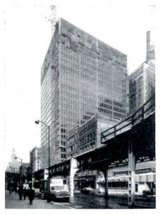
Continental Center in Chicago by Naess and Murphy has columns and spandrel beams faced with welded steel plate
