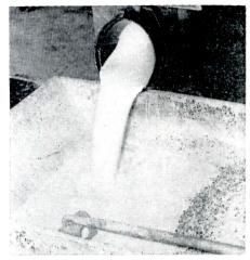
With epoxy terrazzo, resin-curing agent is added to sand and marble chips. To assure a workable mixture some chips are sprinkled on after trowelling
