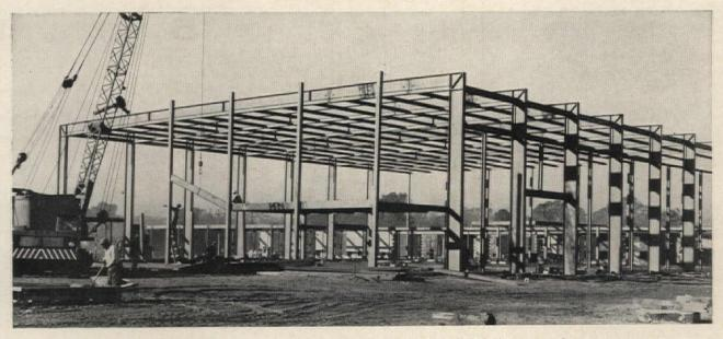
Light weight of plastic-designed steel frame minimized difficulties created by poor subsoil conditions and led to economies in foundation construction.
