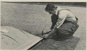
Twin Dome is installed in 15 minutes. Continuous 3" flange is nailed to roof deck, covered with 4 alternating layers of mastic and roofing felt, plus hot tar, gravel.
