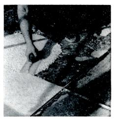
Divider strips are bonded to the sub floor with an epoxy resin-based adhesive
