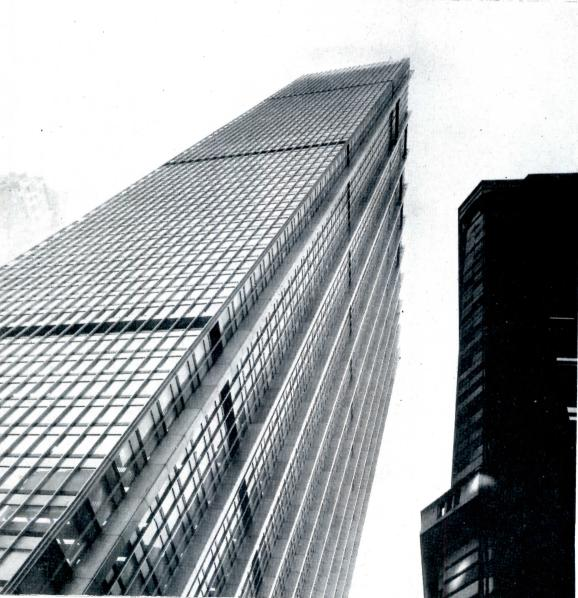
The Chase Manhattan Bank head office building is first skyscraper to the south of Brooklyn Bridge as seen in photo at top of page. Photo made from depth of Wall Street area canyon shows exterior columns which allow uninterrupted interior wall surface
