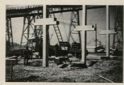
The columns in Huron's 25,000 sq. ft. building are 15" x 16" in cross section by 28'-5" high (two stories).
