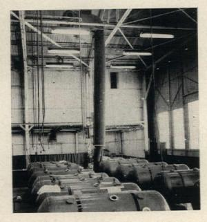
In addition to space heating, Temco, like many other firms, has adapted Janitrol Unit heaters for use in manufacturing or processing. Here, a high velocity heater, located above the lighting fixtures, provides heat through a large fabric duct for use in curing aircraft fuel tanks that are being overhauled.
