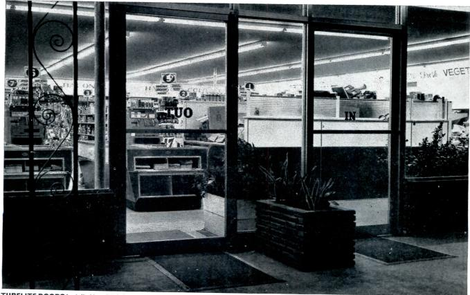
TUBELITE DOORS installed in a PPG Open-Vision front—Harris' Super Market, Waycross, Georgia. PPG's heavy-duty, high-traffic Tubelite entrances have concealed channel type anchors which keep frame seams to a hair line. Door frames have an exclusive interlocking feature that insures rigidity. For shopper convenience, doors are mat operated by PPG's Pittcomatic automatic door opener. Contractor: Business, Inc., Waycross, Georgia.
