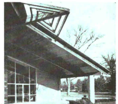
The Holden Museum of Living Reptiles, Detroit Zoological Park, Detroit, Mich. Architects: Charles N. Agree, Inc., Detroit. Rilco laminated wood arches and beams erected by Laco, Inc., Fraser, Mich.
