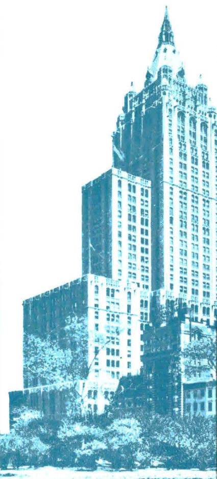
1926 New York Life Insurance Co. Home Office, New York, N. Y. Architect: Cass Gilbert
