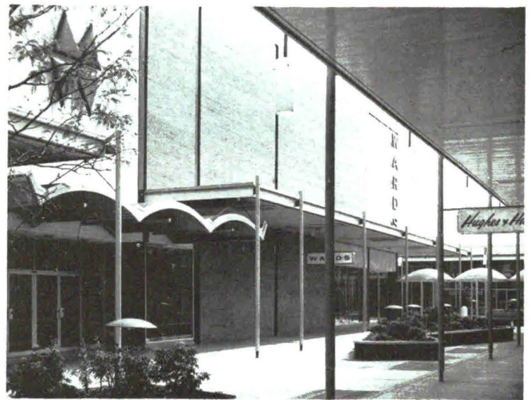
Main entrance mall next to parking
