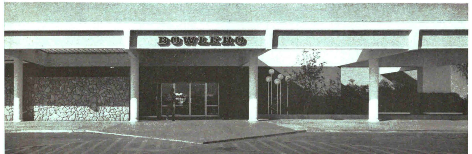
Bowling alley has block walls painted deep rust color, white plaster canopy with yellow tile panels between beams
