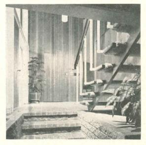
THE STRUCTURE of the house is of wood frame, with exteriors of bearing masonry walls made from split concrete blocks. Aggregates in the blocks are beige colored. Foundations are reinforced concrete. The roof is builtup.
