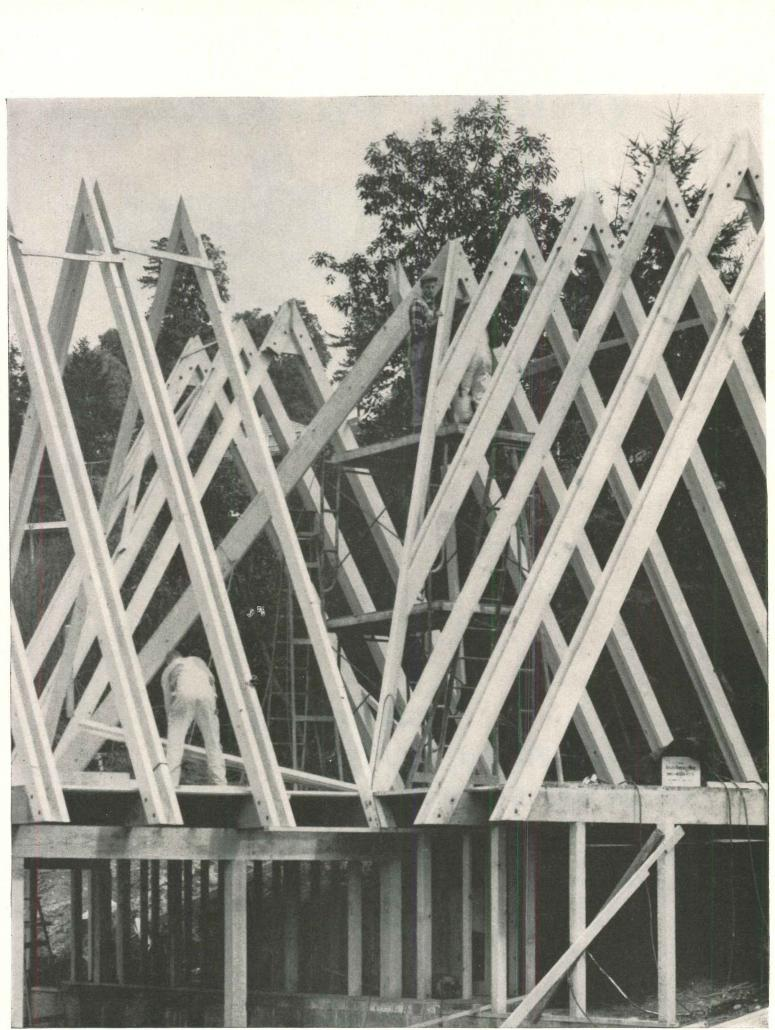
From the ground up, this triangular skeleton tells the story of the A-frame. Sturdy, twin-bolted A-frame beams brace each other to successfully resist the strongest winds, attest to the traditional integrity of wood for minimum maintenance year after year. Dick A. Hill, designer.
