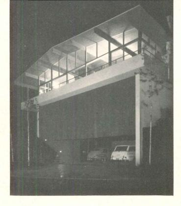
Code restrictions, a steep lot, and a view combined here to effect an unusual design for a hillside house. The local building code requires a five-foot setback at the sides of houses, plus six inches for 100 sq ft over 1,000. A twelvefoot setback is required at the front. The Board of Health further requires a 10-foot setback at the sides for a two-story building. The lot is 60 feet in width, 130 feet deep.
