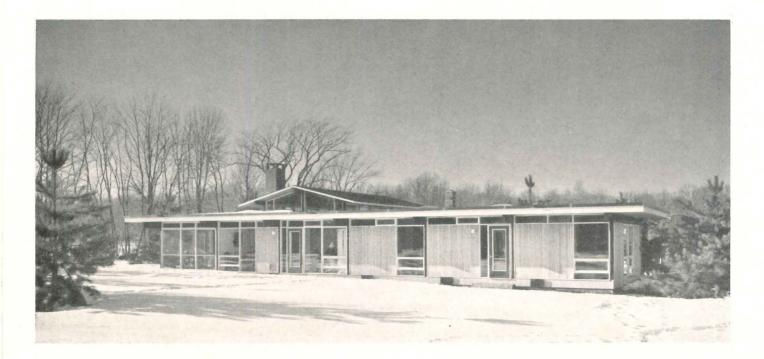
THE STRUCTURE: The frame is wood post and beam on a concrete foundation. Exterior walls are vertical red cedar with a clear finish. Eaves and window sash are painted white. The frame is a darker finish for clear contrast. Ceilings in living areas are 3-in. laminated cedar decking. Roofing is shingle and tar and gravel.
