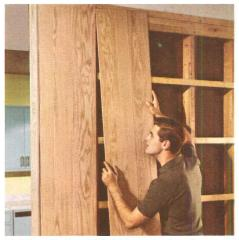
Fast installation. ¼" thick tongued and grooved Random Planks are 16" by 8'... go up with simple clips over furring strips or existing walls.
