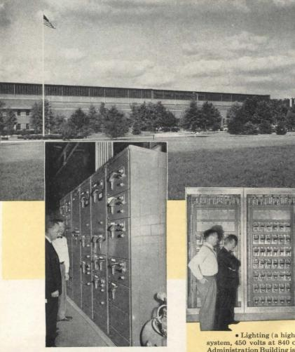
• This Square D control center in the Administration Building includes circuit breaker combination motor starters for the heat pump and air-handling equipment. Heat pump operation is automatically controlled through thermostats and programmed by clock system.
