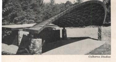
11. The lamella roof of this amphitheater was designed to conform to a cone sector, with the number of lamella joints across the arch, and the angle of intersecting lamellas, remaining constant throughout the length of the roof. This was done by decreasing both the long and short axes of each successive diamond, and inclining the lamella faces in relation to the cone axis so that the stage roof reflects sound to every part of the amphitheater
