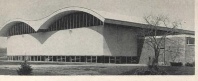
3. This gymnasium is a further example of how the lamella roof may be adapted to achieve an architectural effect. The space is covered by twin barrels, this time of lightweight steel, supported at the center by a beam which leaves the floor unobstructed and also accommodates a folding partition
