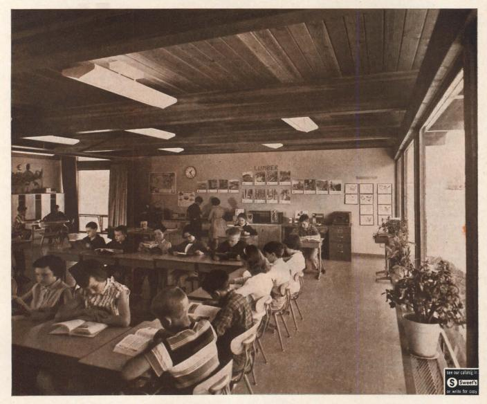
Glued laminated timber beams provide structural framing for a fire-safe school of natural charm while contributing to a saving of 31% in prevailing per-pupil cost of construction.
