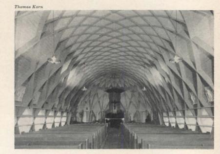
4. The parabolic cross section of the lamella roof for this small church was formed by using a short radius arch in the center section and longer radii for the sides. Since the lamella units for the very short radius would otherwise have required a considerable curved cut, this area was made just half that of the lower portions. This produced a visual division between "roof" and "walls," which was further marked by the installation of sound-absorbing insulation in the smaller ceiling panels
