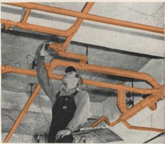
**TESTING A VALVE** on the hot-water supply system. Other copper tube lines in view are part of the sanitary drainage system, ranging in size from  $1\frac{1}{2}$  inches to 4 inches. Because connections are easily made, even in tight quarters, the lines can hug the ceiling.
