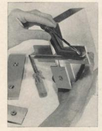
STEP 2—Resilient neoprene seal snaps easily over glass, then gasketed light can be set in place in frame.
