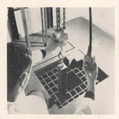
Gamma "garden," the main storage vault for radioisotopes and the highlevel irradiation facility, is a well extending from the first-floor level to the basement level. The 54 storage tubes (one here being sealed by a technician) can hold up to 100,000 curies of Cobalt 60 or equivalent. The 6-ft-sq well in a corner of the building is shielded on the inner sides by shield rooms filled with coarse concrete sand (bulk density: 127 lbs per cu ft)
