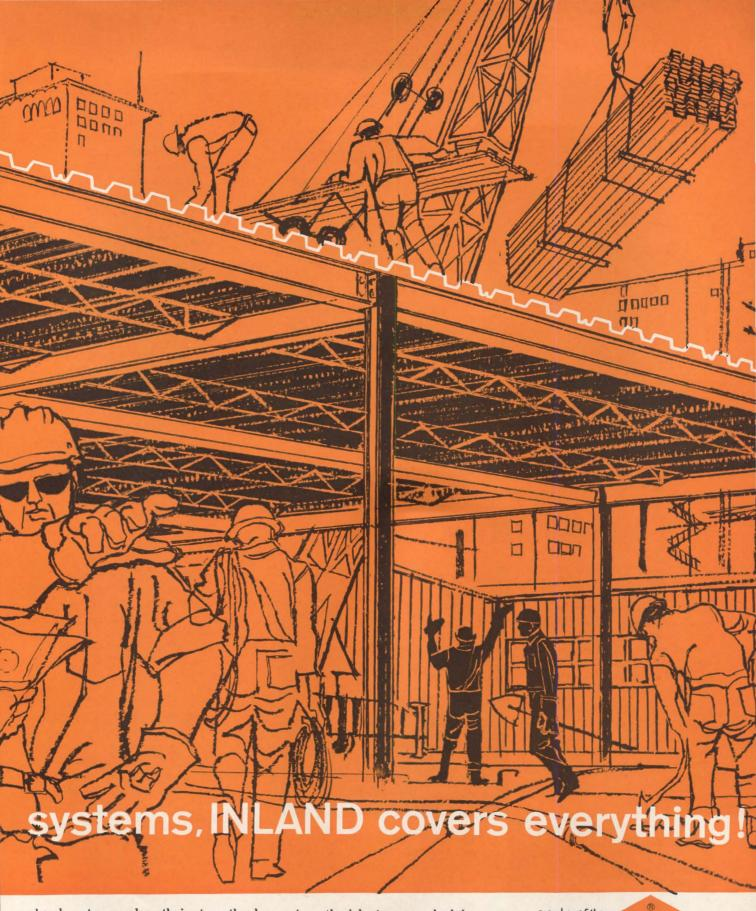
absorb water, nor lose their strength when wet — the job stays on schedule. Types A, B, C, and H decks have the additional advantage of a Bonderized, baked-enamel prime finish that resists on-the-job damage. One field coat of paint on these Inland decks usually does the job of two coats on ordinary decks.
