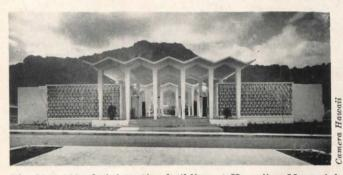
The \$100,000 administration building at Hawaiian Memorial Park on Oahu, opened last month, is of concrete tile block with a folded plate roof and concrete grilles. The structure was designed by Wimberly & Cook Architects, Ltd.; the Highway Construction Co. was general contractor
