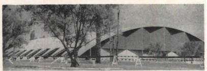
6. Though similar to the conventionally buttressed auditorium shown above, this exhibition hall represents an advance over it in that the need for buttress-type supports was eliminated by pulling the lamella barrel down almost to grade level and scalloping the frame between the low concrete piers. This proved to be doubly advantageous since the considerable reduction in the size of the buttresses cut expenses while the scalloping produced a pleasing esthetic effect
