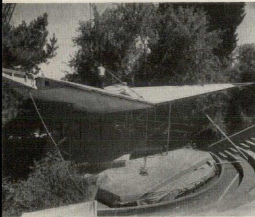
Prefabricated segments of stressed skin plywood are bolted together on the site to form a fanciful four-pointed star that is also strong, lightweight—and economical
