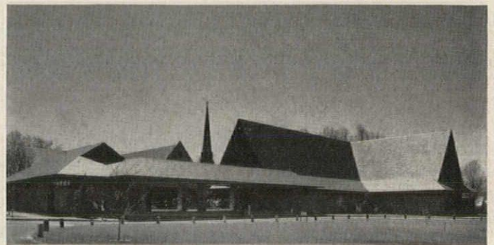
Entrance loggia on north
