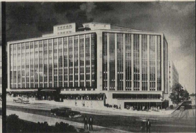
Universal Building, Washington, D. C. - Le Roy Werner, Architect
