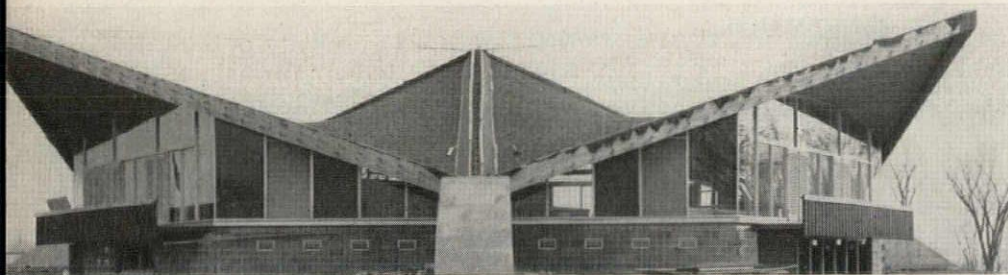
Two-story Massena Country Club is roofed by three hyperbolic paraboloids arranged in a hexagon and supported on concrete piers. Lower walls are masonry; upper walls glass with brightly colored aluminum panels. Sharp definition of each level helps to establish scale
