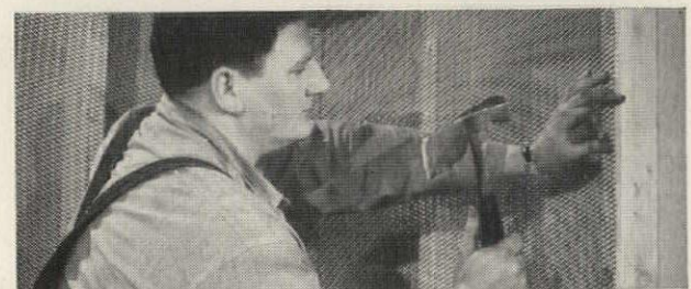
TRUSCON METAL LATH AND ACCESSORIES are specifically designed to simplify and speed construction. Truscon Expanded Corner Bead has heavy shoulders to assure straightness and rigidity. Easier installation, no costly delays. Send coupon.
