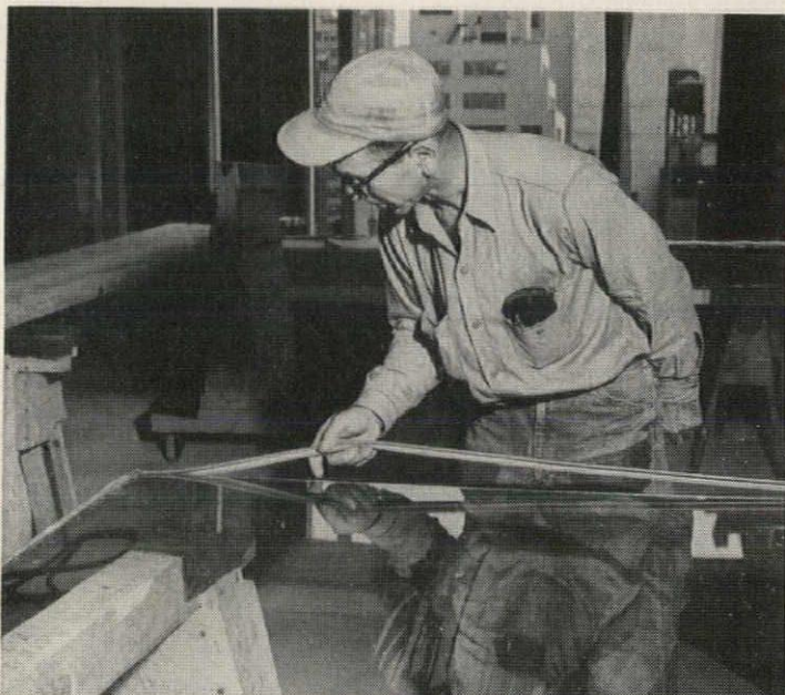
Neoprene gasket with molded corners and U-shaped cross section is quickly installed on the site.
