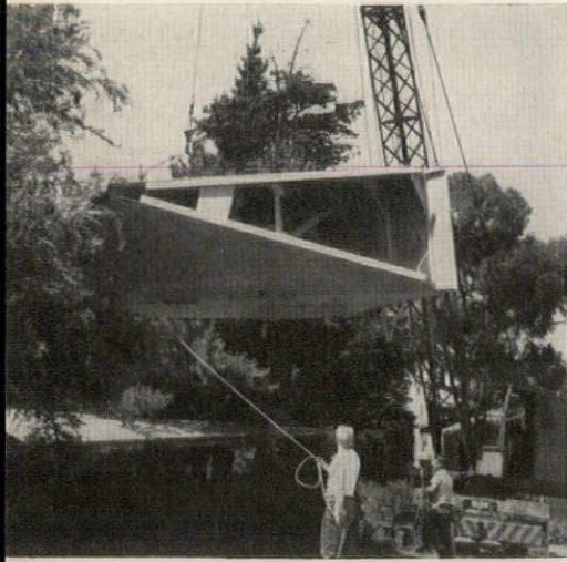
Prefabricated segments of stressed skin plywood are bolted together on the site to form a fanciful four-pointed star that is also strong, lightweight—and economical
