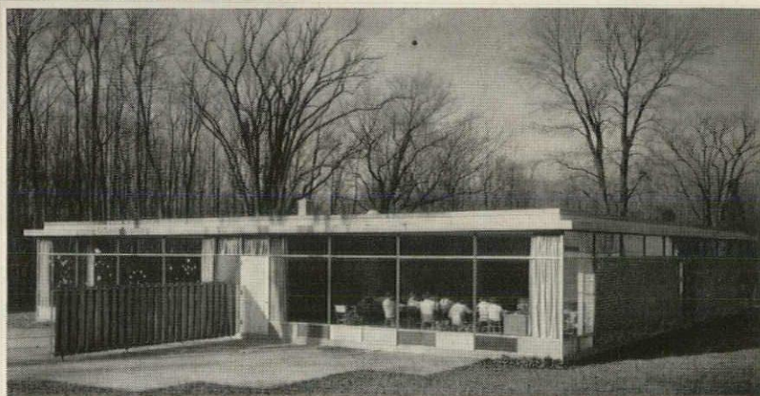
At right: Wilbert Snow Elementary School, Middletown, Conn. Warren H. Asbley, Architect
