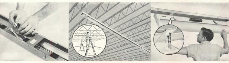
Wire the Uni-Race Branch-circuit wires are laid in the Uni-Race and connection is made at each built-in receptacle. The receptacles will later receive the plug that is built into each fixture. The Uni-Race is U.L. approved as a raceway with a capacity of five No. 8 AWG wires or eleven No. 14 wires.
