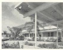
Skipper Motel, Tampa, Florida. For tourist comfort, sound conditioned motels are a necessity in these busy areas. Tectum over concrete beams is featured in this beauty. The second floor is composed of poured concrete on Tectum formboard "left-inplace" as an acoustical ceiling for the first floor. Architects: Goiswald & Reynolds, St. Petersburg.
