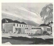
brick façade and curtain walls of glass and cast stone. Framing for wall panels and coping is of alumi-
