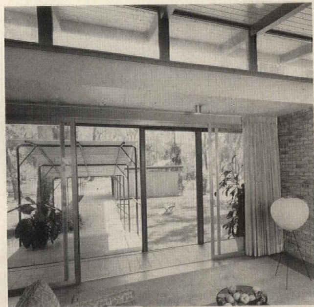
From the living area, the covered walkway is seen as a broad, long, and dramatic promenade. Horizontal roof support for the walkway is achieved by use of (1) cross bars of 1\frac{1}{2} -in. pipe which complete the inverted U-shape of the columns; (2) four lengthwise bars of 1-in. pipe spaced at 2-ft intervals. The porch floor is quarry tile; ceiling is plywood decking on exposed beams. The smooth surface of plaster contrasts with the exposed brick and walnut paneling of the living area.
