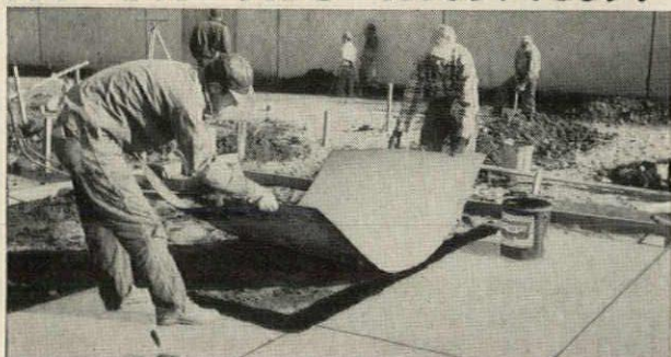
COMPARE the strength... "PM" maintains its permeance rating even after being subjected to the pouring of aggregate, trundling of wheelbarrows and installation foot traffic. Resists rupturing and tearing. How many other materials will perform like this? COMPARE the ease and speed of providing a permanent installation... "PM" may be laid directly over the tamped grade or fill. Ideal for all types of construction; basement, crawl-space and slab-on-grade.
