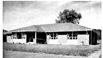
Below: Salvation Army Children's Village, London, Ont.; O. Roy Moore and Company, London, Architects. Photograph shows a typical cottage; overall view is shown in perspective
