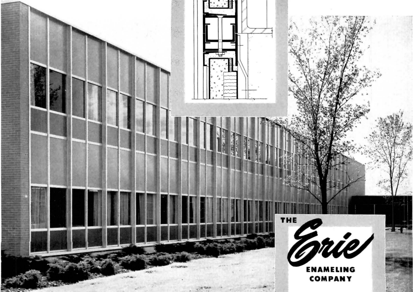
Details at left show a cross section illustrating the special modification of the Erie U-16 Panel used and the method of attachment.
