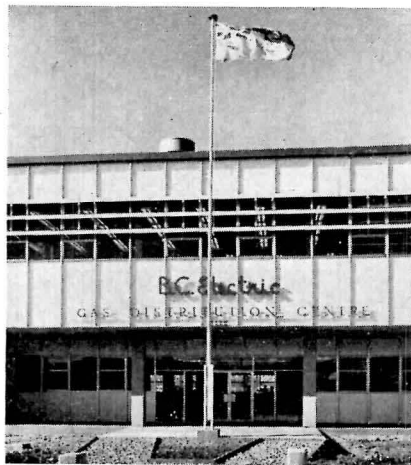
Service headquarters for B.C. Electric's natural gas distribution system, Burnaby; design by B. C. Electric Engineer Company
