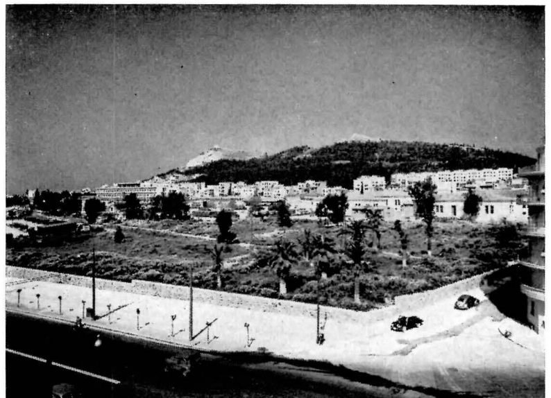
The sloping site on Queen Sophie Avenue
