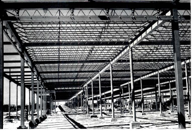
THE TOWN AND COUNTRY PLAZA SHOPPING CENTER, Pensacola, Fla., used 1,825 tons of structural steel, including 448 tons of AmBridge Steel Joists —all fabricated and erected by American Bridge.
