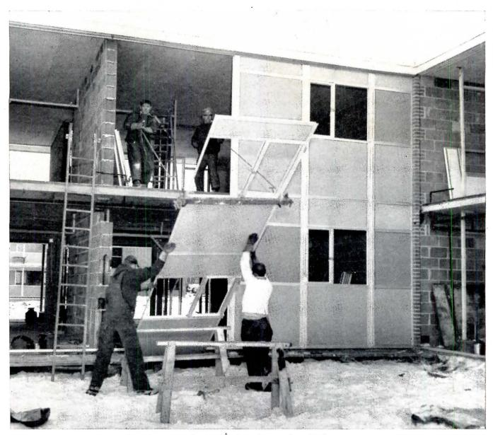
Workmen installing window walls made with Hasko-Struct<sup> $\dagger$ </sup> plastic laminated sandwich panels. Architect is Manson & Carver Associates, General Contractor is Christman Company.
