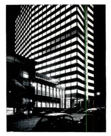
21-story tower is one of three structurally independent components comprising the new Head Office of B.C. Electric. With the one-story assembly block and the threestory sales block, the building covers only two thirds of the site at ground level, one quarter above the third floor. Adjacent is the company's recently completed Dal Grauer Substation (visible at extreme left in photo at right above)
