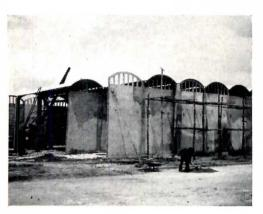
Openings for doors and windows and even glazed skylights as in the shell at right — are formed into the elements as they are cast. To eliminate tie rods and speed erection, column capitals and upper wall sections follow the curvature of the shells they support.
