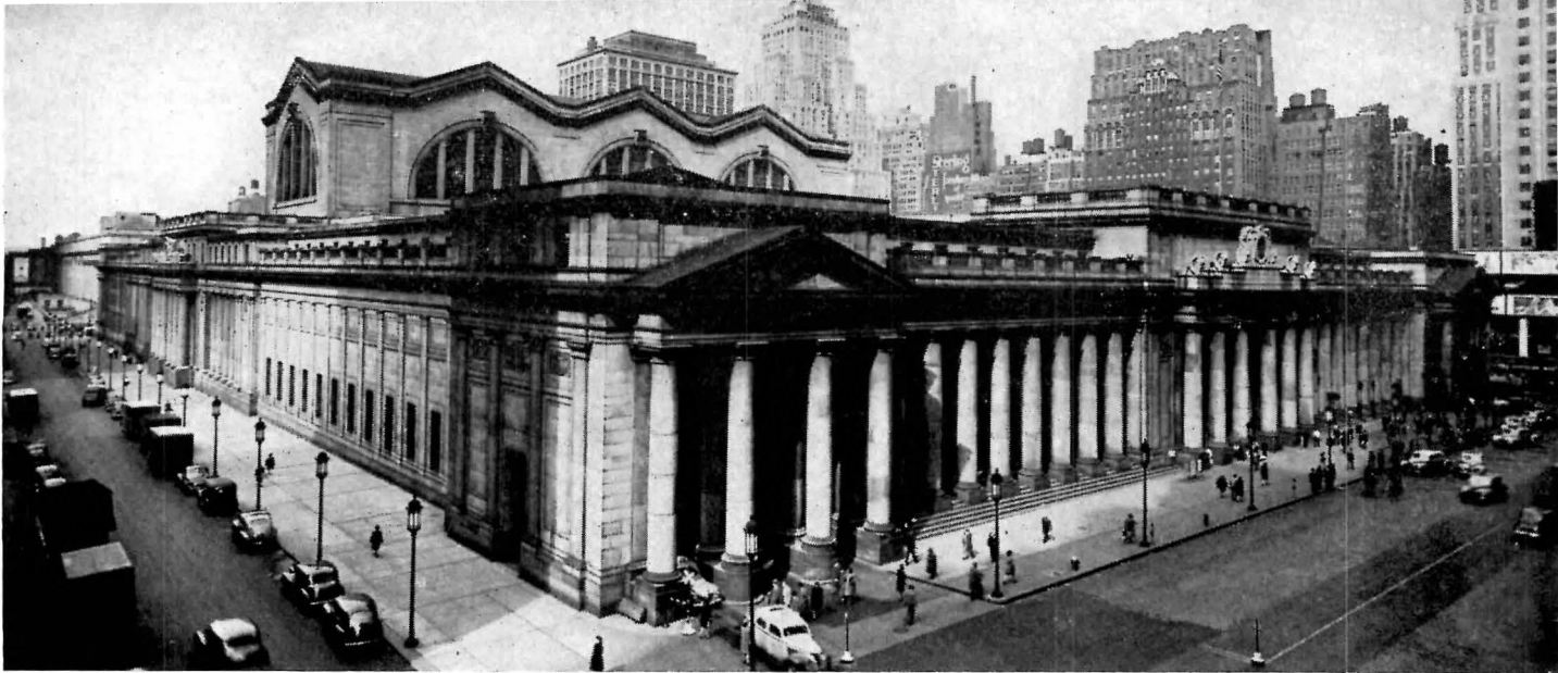
Pennsylvania Station, New York, 1906, McKim, Mead & White. (Tied for twentieth)
