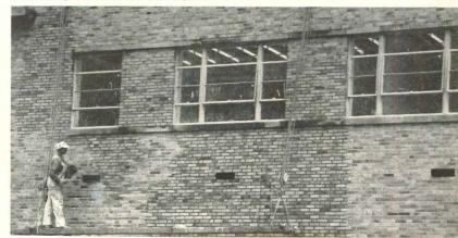
Silicones are applied on large areas by means of a low pressure spray in a flooding action so as to insure thorough treatment
