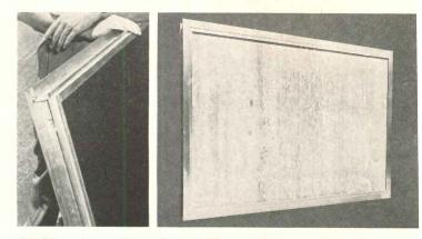
Marble curlain wall panel uses  $\frac{1}{2}$ -in. marble slab backed up by insulation and composition board, all held by an aluminum frame which interlocks with other frames. It weighs 9 lb per sq  $\frac{1}{16}$
