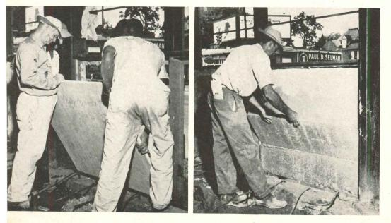
For another marble curtain wall, workmen first insert  $\frac{1}{8}$ -in. slab in spandrel framework, followed by 3-in. rigid insulation; interior has  $\frac{3}{4}$ -in. coat of plaster
