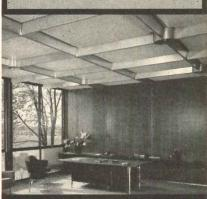
This executive office in the Research Admin-Stration Building, one of seven at the General Motors Technical Center air condi-tioned by Thermotank, shows a typical in-stallation of Thermotank's custom-designed diffusers with integrated sprinkler heads
