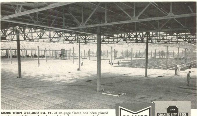
**MORE THAN 318,000 SQ. FI.** of 24-gage Cotar has been placed on the second floor and on fan and transformer rooms of the new Lincoln plant in Novi, Michigan. Cofar deep-corrugated steel units provide main reinforcement. T-wires, welded across corrugations, provide composite temperature reinforcement, mechanical anchorage and shear transfer from concrete to high-strength Cofar steel.
