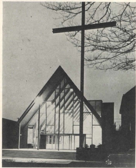
St. Stephen's Episcopal Church, Columbus, Ohio, completed in 1953, Brooks and Coddington, architects
