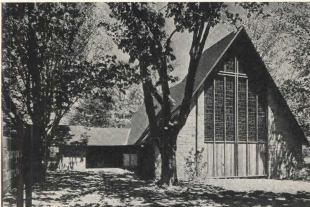
St. George's Episcopal Church, Durham, N. H., completed in 1954, John A. Carler, architect
