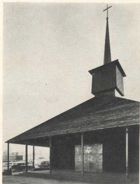
Zion Lutheran Church, Portland, Ore., completed in 1950, Pietro Belluschi, architect
