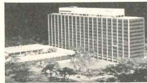
Ford Motor Company Administration Building. 50,000 yds. of Zonolite Plaster machined on. Arch.: Skidmore, Owings & Merrill
