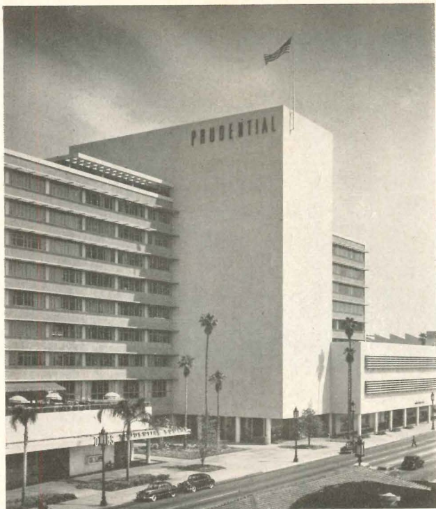
Wellton Becket & Associates, architects
