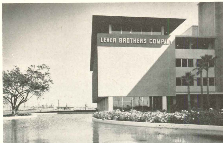
Wellton Becket & Associates, architects
