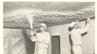
Plaster spurts to a speedy finish on ceilings.
