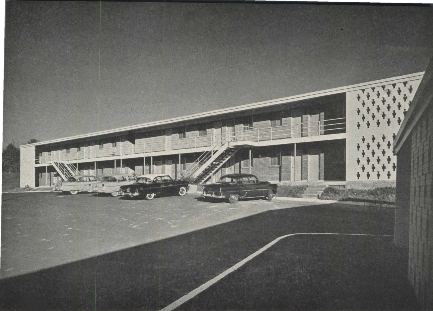
Terrace Motel in Atlanta: two-story bedroom wings directly accessible from paved parking area (J. W. Molitor)
