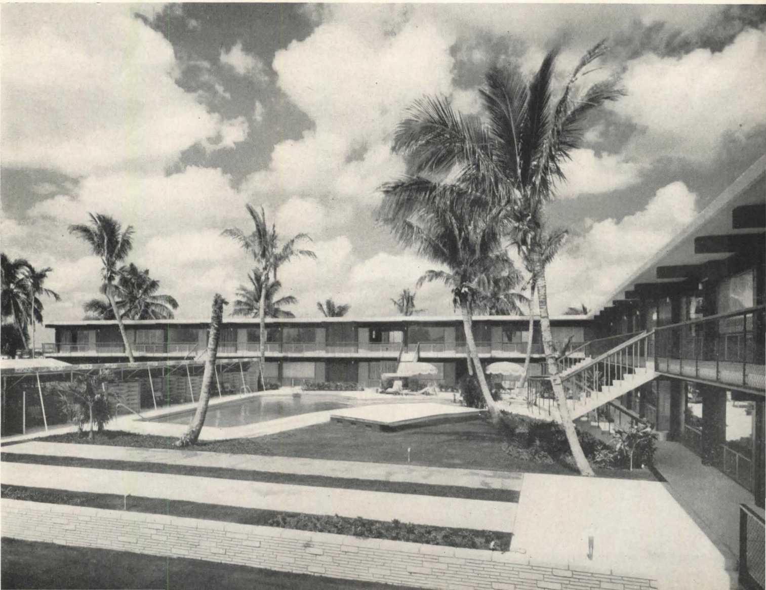
To combat high cost of accommodations at resorts this cooperative motel-apartment-hotel was built recently at Fort Lauderdale, Fla., Robert Hanson, Archt. (Alexandre Georges)
