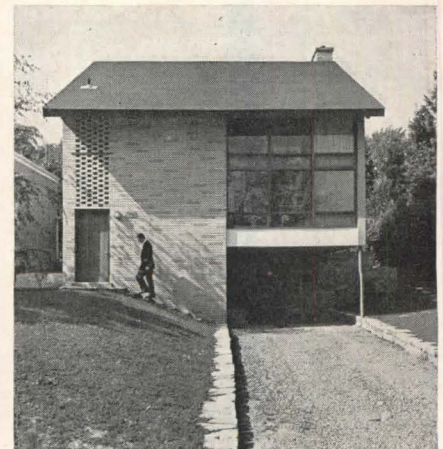
itects Blackwell, Craig & Zeidler, was termed "a triumph in the adaptation to unfavorable site conditions"
