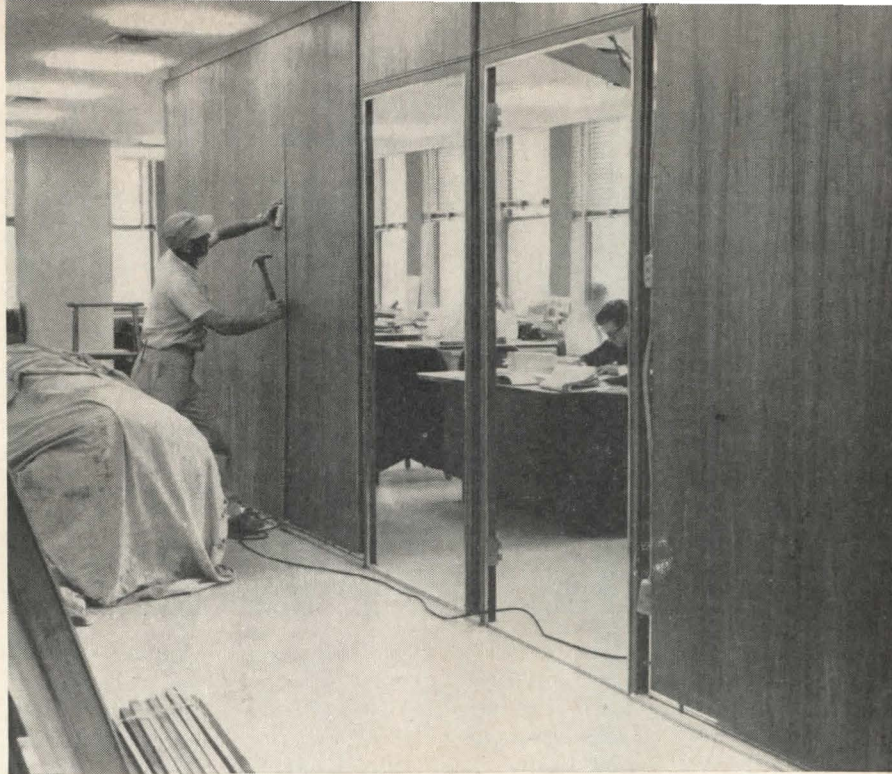
PARTITIONS ARE INSTALLED without costly interruption of regular office routine. Workman is shown installing section of Weldwood Movable Partition; completed corridor is shown at left.
