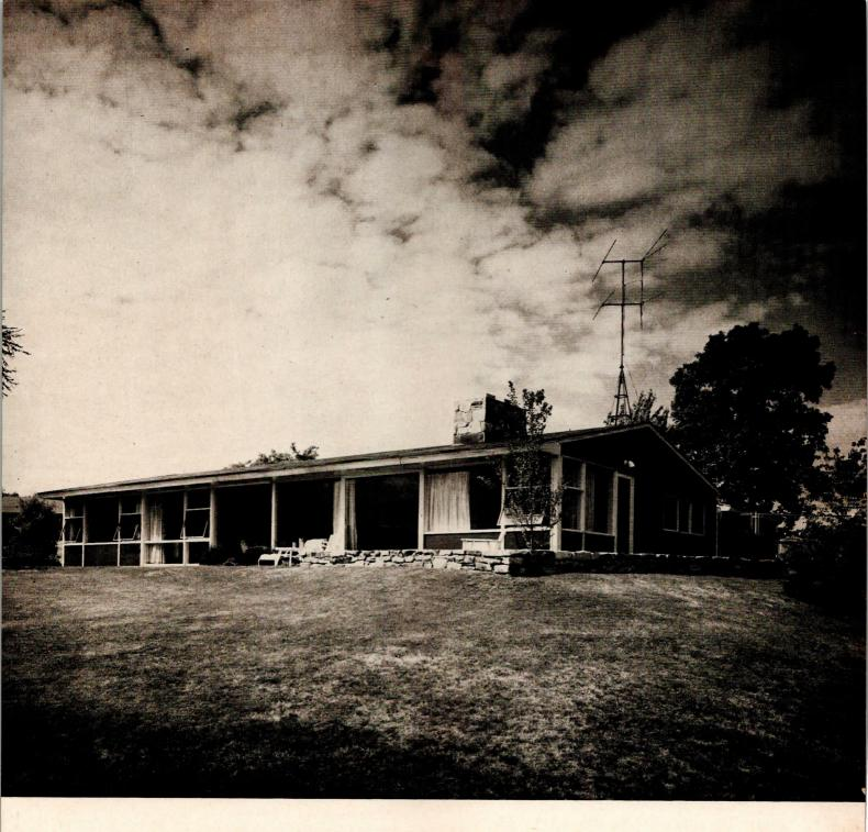
Site Relationship. Site is large, with a long gradual slope at rear which low pitch of roof echoes; living room has floor-to-ceiling glass wall which extends room to far corner of site. Materials. Vertical T&G siding and painted (red) plywood panels on exterior; concrete floors
