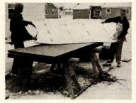
the extra length protrudes and seals any openings at the bottom plate. Reflective Kimsul "48" Sheathing Blanket is stapled to the sheathing board, which
