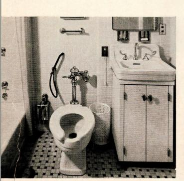
Patient's bathroom with Crane Whirlton siphon jet closet with integral bedpan lugs. Crane bedpan cleansing fixture, Neuday porcelain enamel bath, and Norwich vitreous china lavatory.
