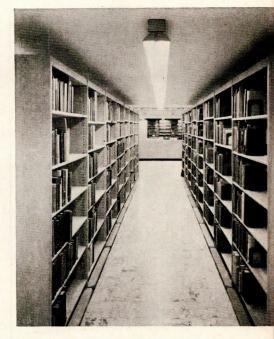
From the top to the bottom shelves in these stacks an ample 30 to 40 ft. candles allows swift and easy identification of any volume. A perfect application of Day-Brite's standard single-lamp STRIP units with symmetric polished alzak reflectors.
