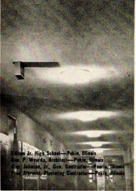
Specify CORALUX — the perlite accoustical plaster — whenever attractive, sound-abosrbent, fireproof surfaces are required for ceilings and upper walls! CORALUX is pre-mixed, smooth - working, non - setting, lightweight (only 9 oz. p.s.f., ½" thick) and non-combustible. Can be troweled or machine applied over old or new surfaces economically. Actually costs less than tiles with comparable acoustical control factors. Write for your file copy of our latest CORALUX Acoustical Plaster bulletin.
