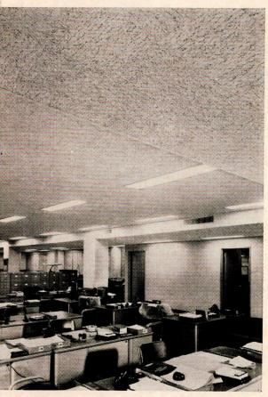
Mistakes caused by distracting noise are reduced in this modern office area. Noise-muffling Travertone soaks up disturbing noise, prevents the clatter of business machines from building to distracting levels.
