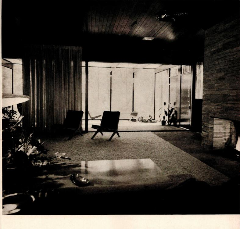
Warm Materials. Construction is wood frame on concrete slab with exterior siding of T&G redwood in contrasting vertical and horizontal treatments; in living area ceilings are redwood, walls are white plastered; chimney is flagstone, as are floors in entry and screened porch
