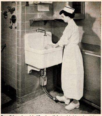
Crane Yale wash-up sink of Duraclay with foot pedal mixing valve which may be elevated to clean the floor. At left of picture, is pre-natal shower with thermostatic control valve and dial thermometer volume control. Hose and shampoo attachment. Vacuum breaker safeguards sterile water supply.
