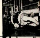
Cold Generator is the packaged water chiller for smaller installations. Engineered, built, tested and refrigerant-charged at factory. 10 to 100 tons.
