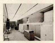
· A luminous ceiling of white translucent, corrugated vinyl rests on extruded aluminum channels under Pittsburgh fluorescent or slimline strips. The "Luma-Ceiling" can also be installed with an auxiliary spun-glass acoustical baffle for sound absorption. The installation shown above is the Paramount Garment Shop in Philadelphia. Pittsburgh Reflector Co., 403 Oliver Bldg., Pittsburgh 22, Pa.
