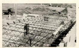
Truscon "O-T" Steel Joists for floor and roof supports. They are light, strong, and fire-resistant. Easy to handle, they lessen the time and labor required for erection, save material in supporting framework and foundations.
