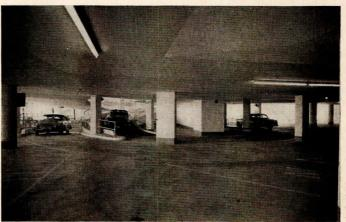
Since garage is self-service, easy grade on ramps which patrons use is essential: Downtown Center's ramps are wide, have 9.5 per cent grade. Nine floors, basement and roof provide 1100 parking spaces
