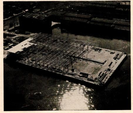
NEW PIER IN EAST BOSTON HARBOR—Shown at left under construction is Pier 1 in East Boston Harbor. This \$9½ million marine terminal and warehouse is 340 ft by 580 ft, and contains over 1600 tons of Bethlehem Structural Shapes. Besides regular pier facilities and tremendous storage capacity, the warehouse contains facilities for pumping liquid cargoes directly from ship to tank car.
