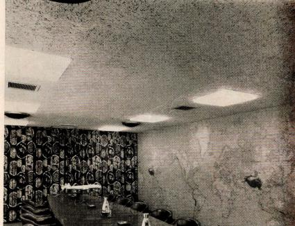
Completely incombustible, Travertone meets all fire-safety regulations. Its handsomely fissured surface resembles travertine marble and can be washed or repainted as often as desired without impairing its acoustical effectiveness.
