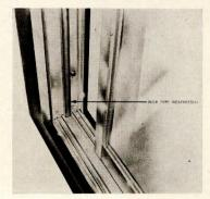
Aluminum sliding glass doors that have a two-piece sill allow installation of a sub-sill before laying of the finished floor. The sill track is installed after all work is completed, so that there is no damage to the track. Bulb-type weather-seal is used in the jamb frame, and double pile-type in the bottom rail. Ludman Corp., North Miami, Fla.
