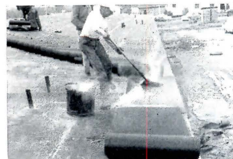
Ideal Base for Built-up Roof. This deck is ideal from two standpoints — a good deck for the roofer to work on—more important, throughout the life of the building, it is an inorganic permanent base for the built-up roof.
