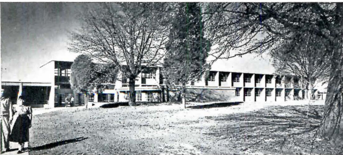
Top Award: (above) West Charlotte High School, Charlotte, N. C.; architects Graves and Toy, Charlotte. Jury's comment: "Well composed campus type plan, designed on a good scale for youth"
