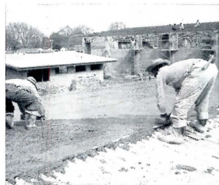
Permanent, Incombustible Roof Deck is provided by cast-in-place slab. When concrete is screeded to depth of 2 1/2"-3", load tests show safety factors of 6 to 8 for finished deck.
