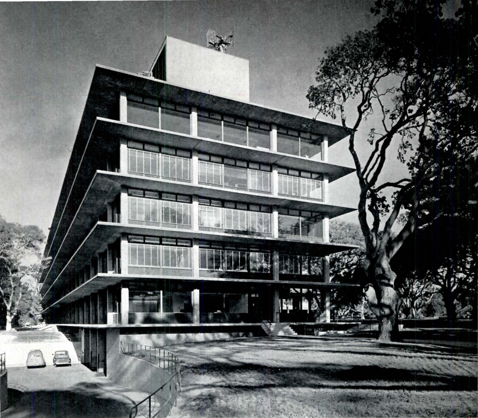
Cantilevered canopies continue around building as expression of flat plate construction, provide sun control, ease building maintenance; structure is dramatically revealed at night. Covered walk (below, right) between lab sciences and auditorium bridges sunken terrace outside cafeteria
