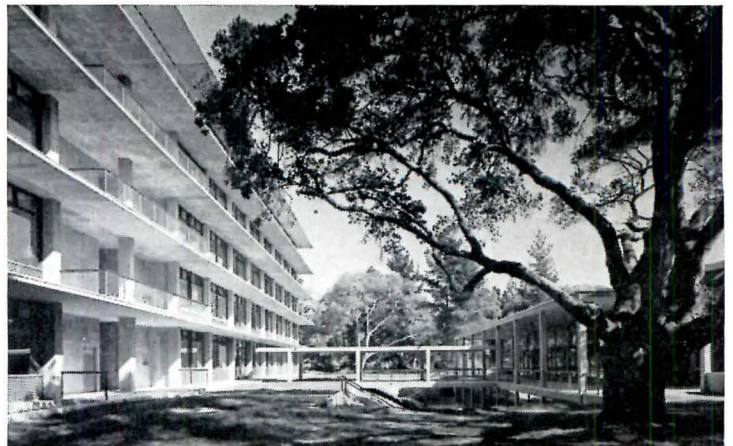
Cantilevered canopies continue around building as expression of flat plate construction, provide sun control, ease building maintenance; structure is dramatically revealed at night. Covered walk (below, right) between lab sciences and auditorium bridges sunken terrace outside cafeteria
