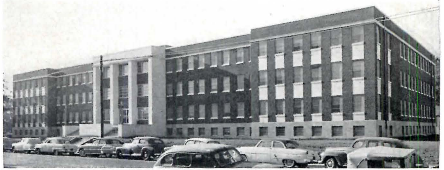
Men's dormitory for Baylor University (Texas) accommodates 340, cost $700,000. Area per occupant, 176 sq ft; study-bedroom, 107 sq ft; toilet-shower, 10 sq ft. Architects: Easterwood & Easterwood
