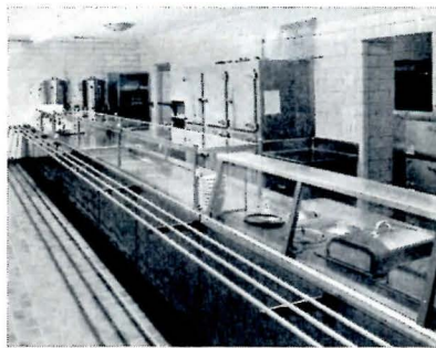
Warm foods are passed through warming compartments to steam table at right; salads and fruits through refrigerated compartments in South Quadrangle
