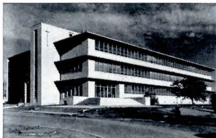
TEXAS. Fenestra Steel Windows in the Science Hall at St. Mary's University, San Antonio, Texas. Architect: Julian & White, San Antonio. Contractor: Lynn & Morse, San Antonio, Texas.
