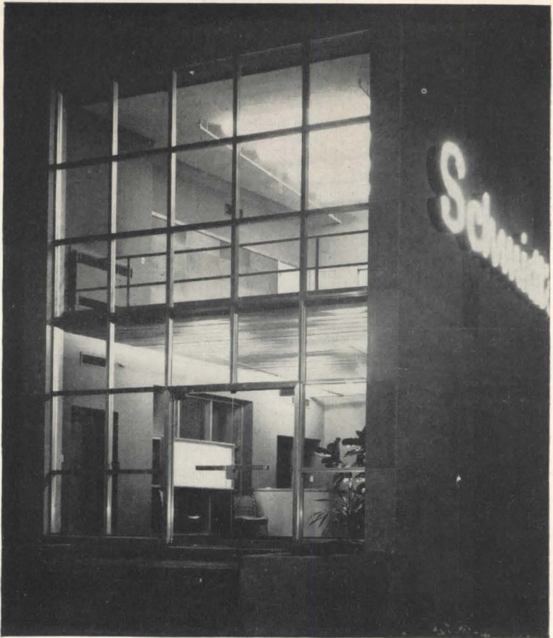
THIS INTERESTING entrance at the Schmidt Provision Company, Toledo, Ohio, is completely walled with Pittsburgh Plate Glass (approximately 20 ft. wide and 20 ft. high—running from the floor to the ceiling). It is set in Pittco De Luxe Sash No. 12 C and divided with horizontal and vertical mullions of No. 24 CTC. The doorway itself is a standard Pittsburgh Doorway, Style No. 16. Architect: Karl B. Hoke, Toledo, Ohio.
