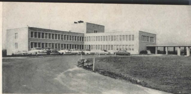
St. Clair Hospital, Mt. Lebanon Township, Pa., serving the growing South Hills area has 116 beds—cost $1.34 million. Steeltex used in all floors. Kuhn & Newcomer, Architects. R. A. Zern, Structural Engineer. H. Busse, Contractor.
