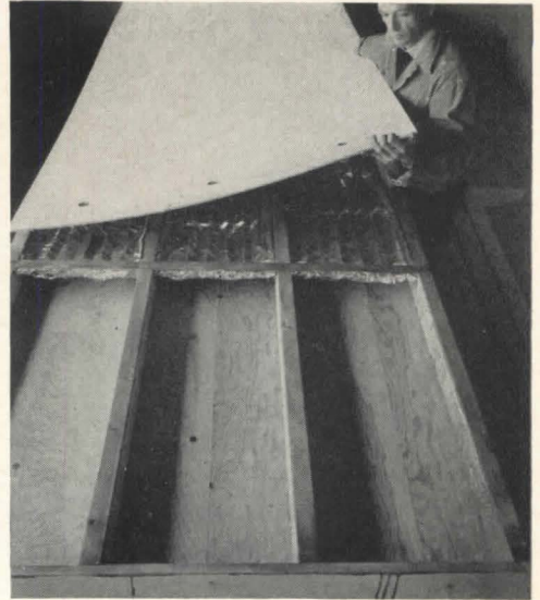
Stressed-skin roof panels, 4 by 16 ft., of fir plywood pressure-glued to 2x4's, are shop-assembled for installation in Carl Koch's Techbuilt house (left). Note aluminum foil insulation which has been inserted between the plywood skins
