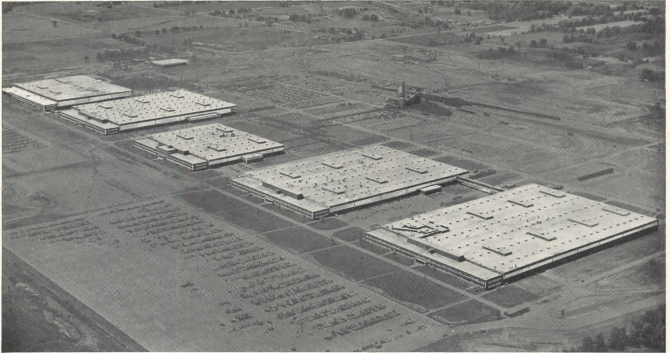
3 MILLION SQUARE FEET OF FIBERGLAS ROOF INSULATION —General Electric's Appliance Park, Louisville, Kentucky. Architect: Albert Kahn & Assoc., Detroit. Gen. Cont'r: Turner-Struck Const. Co., Buechle, Ky. Roofers: Brown and Kerr Roofing Co., Chicago; Schreiber Roofing, Detroit, Mich.
