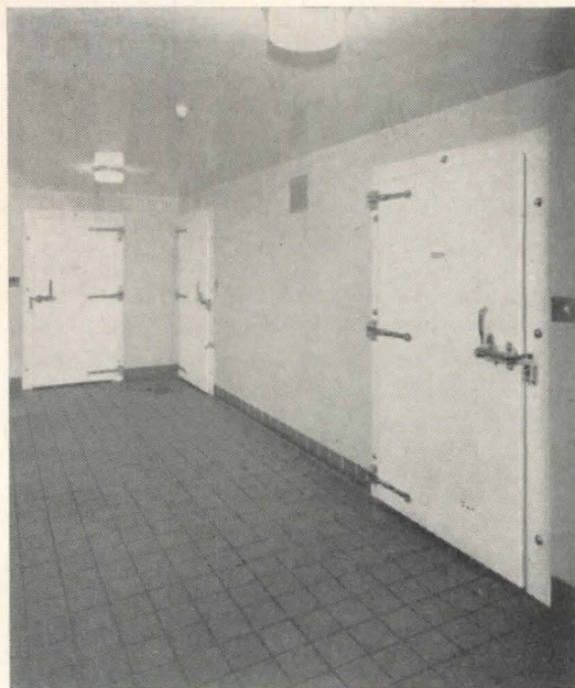
ATTRACTIVE APPEARANCE . . . Glistening white enamel over galvanized metal cladding and chrome hardware. Match harmoniously with the sanitary walls. The three doors above (l. to r.) lead to: cold cuts room; vegetable and fruit room; meat room.
