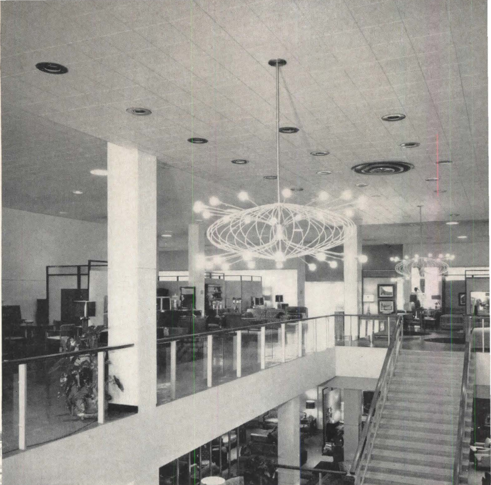
Over the stairway in the Robinson Furniture store, a noise-muffling ceiling of Full Random Cushiontone helps keep disturbing noise from traveling through the open stair well. With perforations spaced at random over the face of each Cushiontone tile, the finished ceiling effect is truly non-directional.
