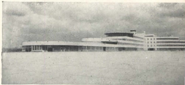
Mammoth decks in this fabulous $10-million terminal building at $42-million Greater Pittsburgh Airport, were poured on Steeltex Floor Lath. Last year 2.5-million people including travelers spent $20 million at ticket counters, restaurants, nightclub, theater, hotel and shops. Joseph Hoover, Architect. Leland Cook, Structural Engineer. Dick Construction Co., Contractors.
