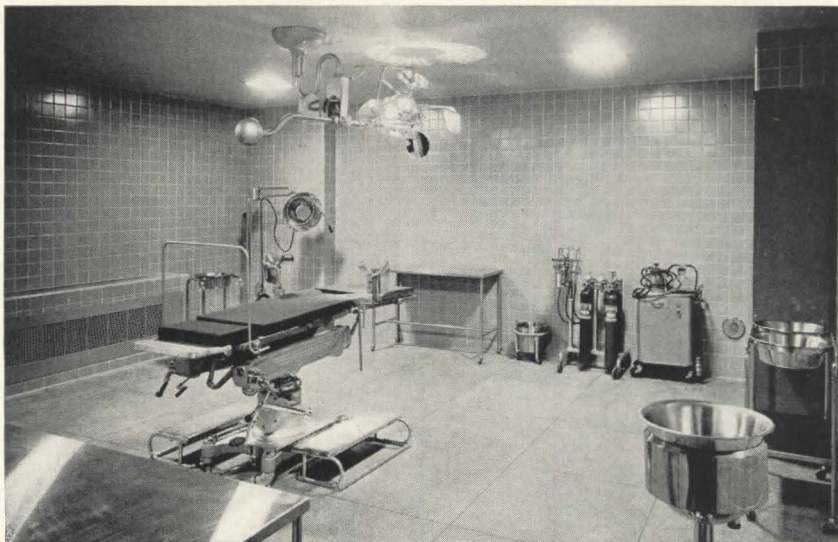
One of the major operating rooms
