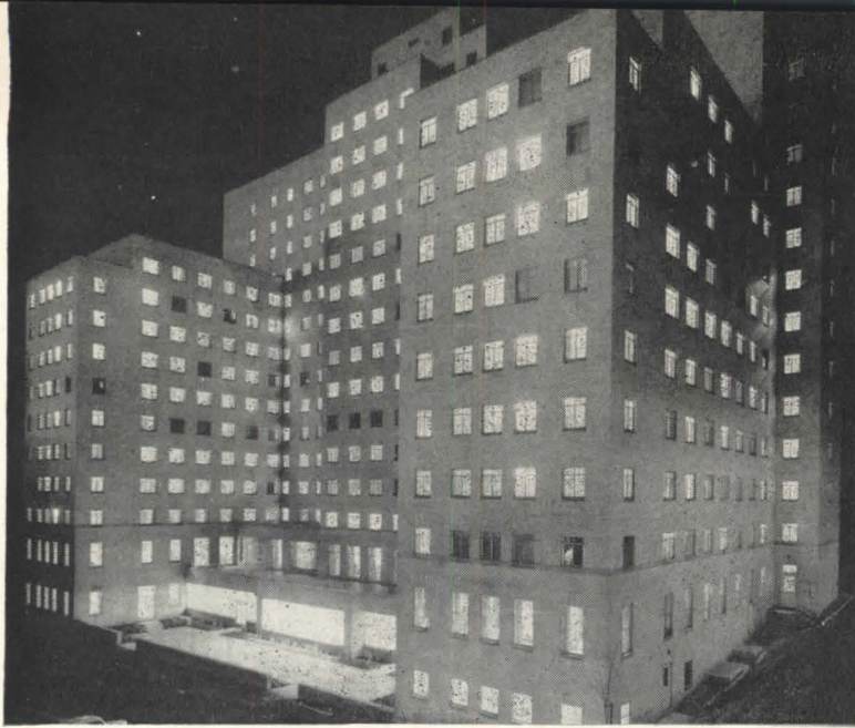
The $3.5-million nurses home at University of Pittsburgh towers 14 stories, completely air conditioned, contains library, recreation room, reception rooms, cafeteria seating 400—comfortable living quarters for 600. Steeltex in upper floors. Ingham, Boyd & Pratt, Architects. Trimble Company, Contractors.
