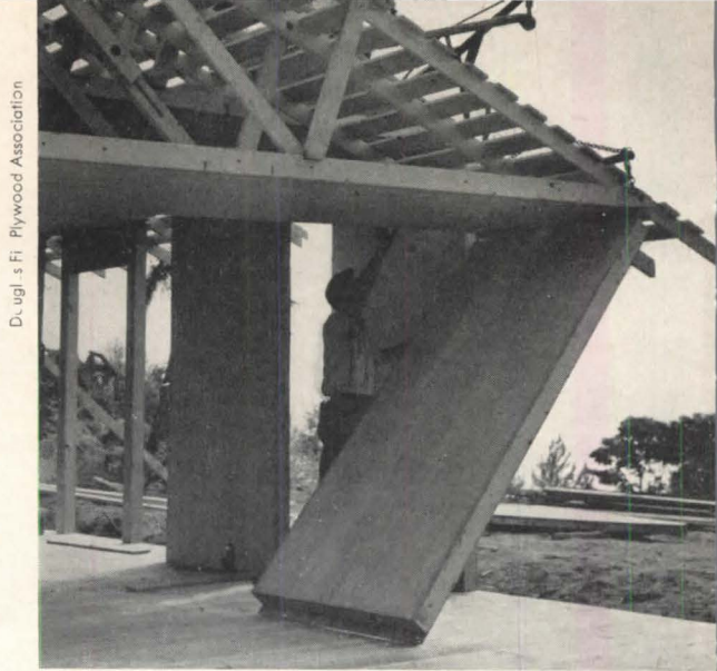
Left: Typical stressed-skin panel. Right: Stressed-skin wall panel which is hinged to ceiling panel and swings into position as roof section of three wood trusses is hoisted into position for a house designed by John Graham, Seattle architect
