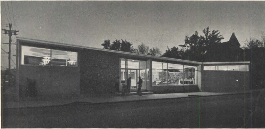
Open, inviting character of building reflects informality of small Western town
