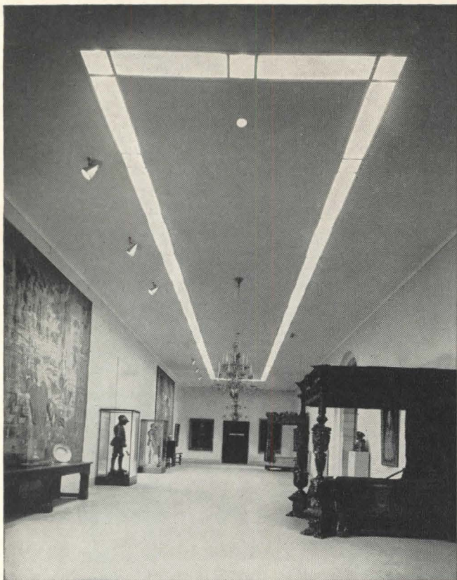
Incandescent and fluorescent light are combined to illuminate this exhibit of 16th and 17th Century English Art in glare-free, shadow-free lighting. Water-white curved lens panels and lenslites blend the two types of light.
