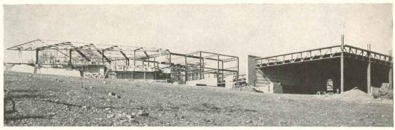
Structure follows slope with minimum excavation. Photo below: at left is chapel; right, side entrance to narthex
