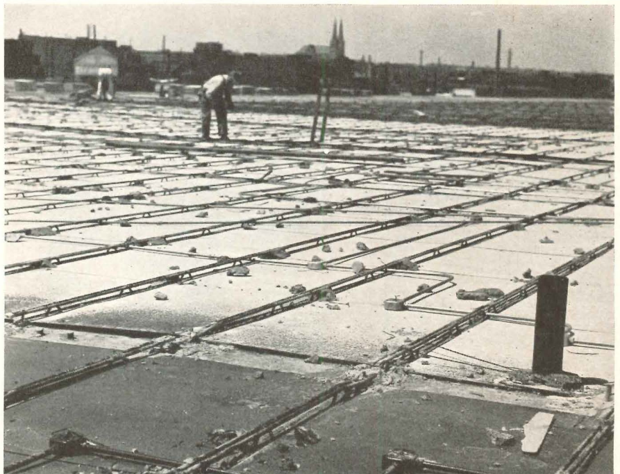
Above: exposed steel bars of concrete joists are welded to plates in wall panels. These bars, also welded to joist stirrups, project up into concrete roof slab to tie slab to frame. Right: asbestos cement sheets act as forms for vermiculite concrete roof fill. All conduit is in roof slab
