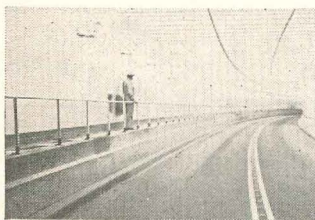
Almost one mile of Seaporcel Porcelain Enamel Flush Type Patented Handrails line the tunnel. Designed with concealed internal fastenings, completely prefit, readily installed and eliminating on-the-job welding.
