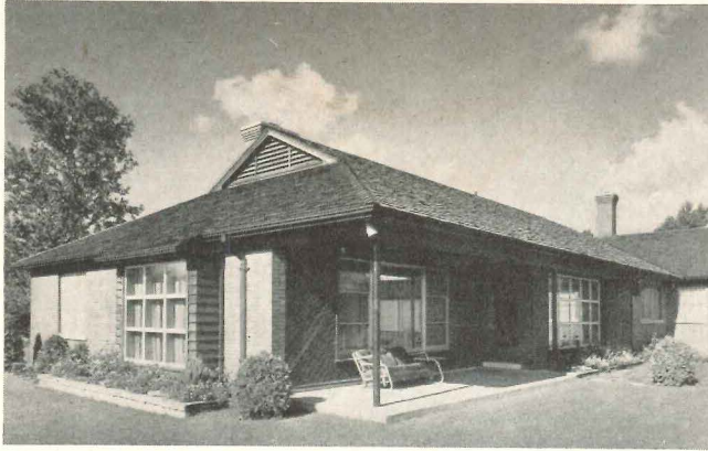
White & Hastings of London, Ont., were architects for the Wallace Weinstein residence in London
