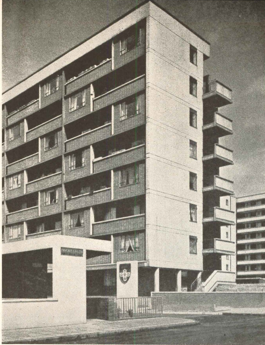
Above: "box-frame" construction was recently used for a series of apartment buildings in London, England. (Photo: The Architectural Review, Oct. 1952)
