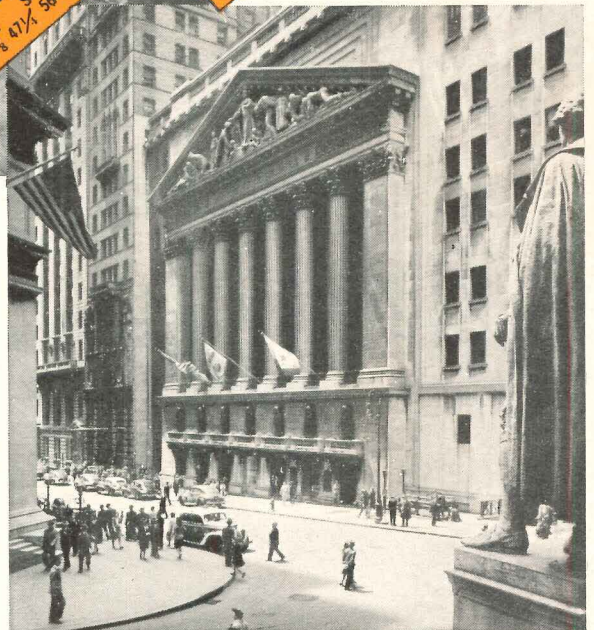
Consulting Engineer present air conditioning system: Charles S. Leopold
