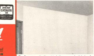
The FIRESTOP wall adjacent to bathroom remains intact and undamaged. On other adjacent walls the intense heat blackened the nailheads, but FIRESTOP Bestwall remained undamaged.
