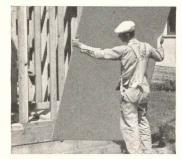
BILDRITE SHEATHING goes up faster, easier. Cuts application time at least 25%. 4-foot sheets have twice the bracing strength of horizontally-applied wood sheathing thus save corner-bracing. Waterproofed throughout—eliminates need for building paper. No waste.
