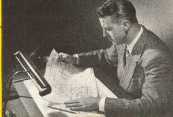
The direct-process prints and blueprints received from vendors are reproduced on Autopositive Paper when extra copies are needed for the drafting room or shop. Deletions and additions can be made readily on Autopositive intermediates ... saving drafting time.
