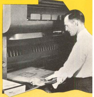
How positive photographic intermediates are produced. Kodagraph Autopositive Paper is exposed in Sikorsky's direct-process machine . . . processed in standard photographic solutions. No negative step... no darkroom handling – a revolutionary, economical operation that speeds print service to all departments!
