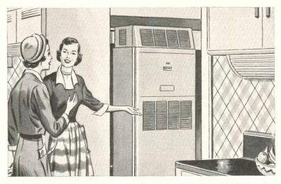
With other heating systems – such as radiant heating – Frigidaire Air Conditioner is installed in a concealed central location. Short ducts lead to the rooms, and cooling for each may be controlled as desired. This plan is ideal for single-story homes.
