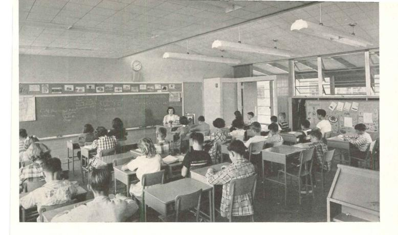
Every classroom has window sill at height suitable for age group. Several scale models were made of typical classroom sections and tested with light meters to assure uniform light intensity throughout the room
