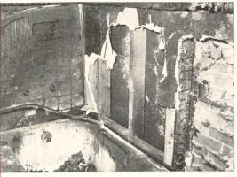
Right foreground shows section where firemen broke through FIRESTOP during blaze. Charred side of wooden stud is the result. Then compare remaining undamaged studs between the FIRESTOP wallboards. Wallboards were broken away after fire to show undamaged condition.
