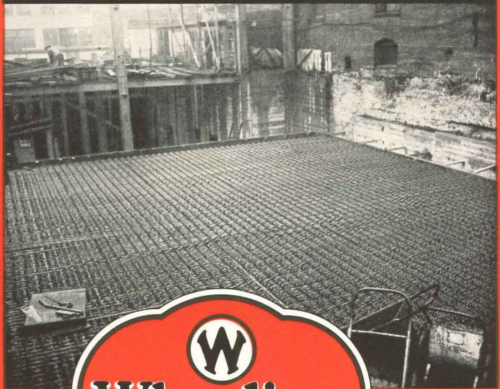
In the roof view, note the relatively long spans made possible by Steelcrete's lateral stiffness.
