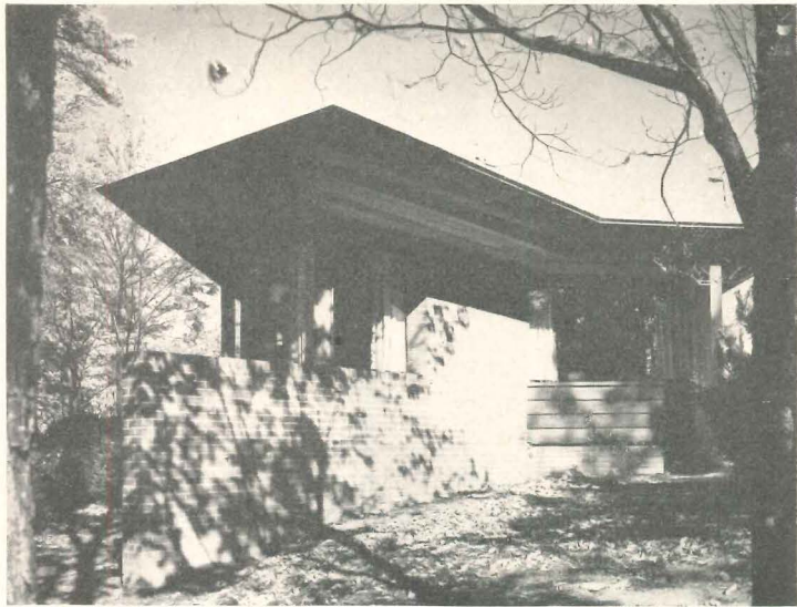
End of bedroom wing, seen from outside (above) and inside (below). Bottom of page: living room terrace. Fore-shortened wall is same shown on p. 122
