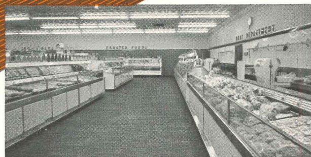
Heat from these display cases is disposed of through tubing buried below basement floor.
