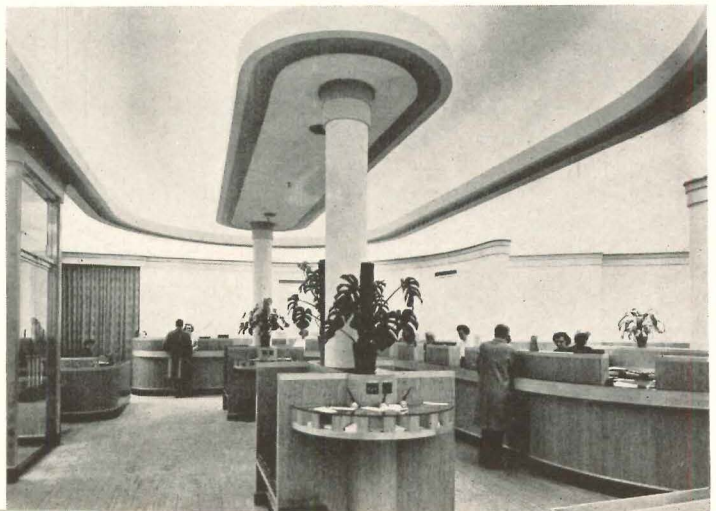
Bank lighting layout considers shape of room in combining indirect cove illumination with an egg-crate ceiling which has a higher intensity for work areas
