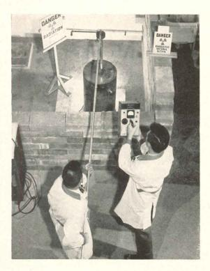
A technician stands behind a barrier and uses a long pole to lower a sample by remote control. The health physicist (right) uses a survey meter to make sure that the technician is not exposed to dangerous amounts of radiation parts: one "cold," and one "warm." The warm process waste would then need to be retained in a bottle or tank until analysis would indicate what manner of disposal would be considered necessary.
