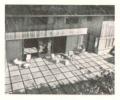
Upper or rear lanai is paved with concrete blocks using a coral aggregate; joints are planted with a Japanese moss grass. Wires above are to carry vines to provide needed shade in middle of day
