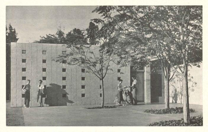
Known as the ''Y'' youth center, this activities building was constructed at  $V_3$  to  $V_2$  the comparable cost of conventional Y buildings in California. Modular construction, elimination of much plaster, articulation of plan and similar factors are credited with keeping cost to \$29,000
