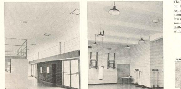
The lobby, gymnasium, and other rooms of St. Mary's are sound conditioned with Armstrong's Cushiontone, a wood fiber acoustical material. It was chosen for its low cost, high sound absorption, and clean, smart appearance. Cushiontone has neatly drilled perforations, and its washable white paint finish is high in light reflection.
