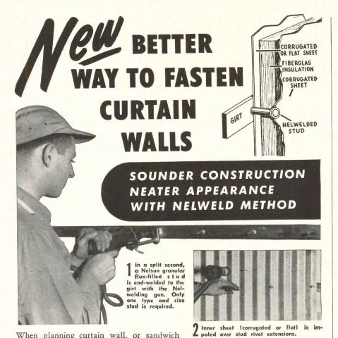
When planning curtain wall, or sandwich type, construction, it will pay you to investigate and specify the Nelweld method of fastening. Used on such outstanding projects as the new Fairless steel plant, Morrisville, Pa., and the Lincoln Electric building, Cleveland, this method provides these advantages:
