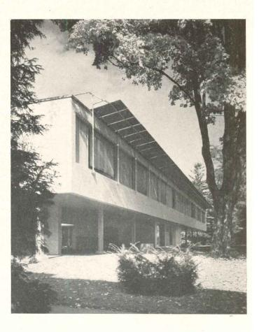
The fun of structural things in tension here comes out in a cable stabilizer for the pipe-supported sunshades. Shade itself is sections of corrugated asbestos cement, with small spaces between sections to make light stripes across the building
