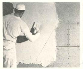
Bonding Power of plaster to LOK-JOINT LATH is more than *twice* that required by the commercial standard for structural fiber board. Exclusive rigid metal "Loks" stop annoying "yield-and snap-back" at joints. Large units lay up quickly; save time.
