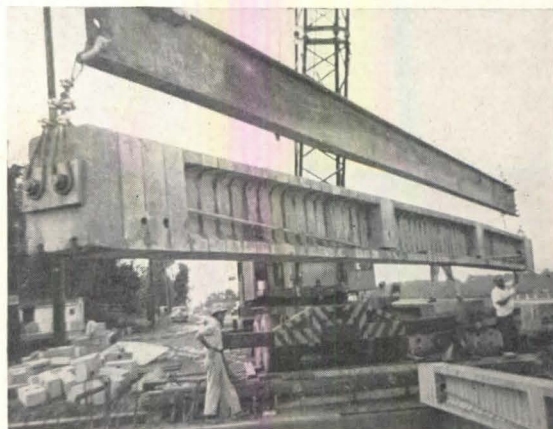
Below: machine-made blocks shown at left were assembled into prestressed girders for a highway bridge near Detroit, Michigan
