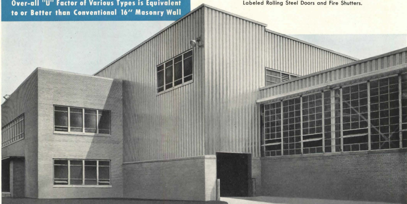
Mahon Insulated Metal Walls employed in construction of a new plant for Ford Motor Company in Cleveland, Ohio. F. A. Fairbrother and Geo. H. Miehl Architects-Engineers. Albert Kahn Associated Architects and Engineers, Inc., Consultants. H. K. Ferguson Company, General Contractors.
