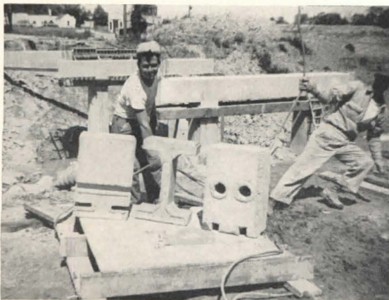
Below: machine-made blocks shown at left were assembled into prestressed girders for a highway bridge near Detroit, Michigan
