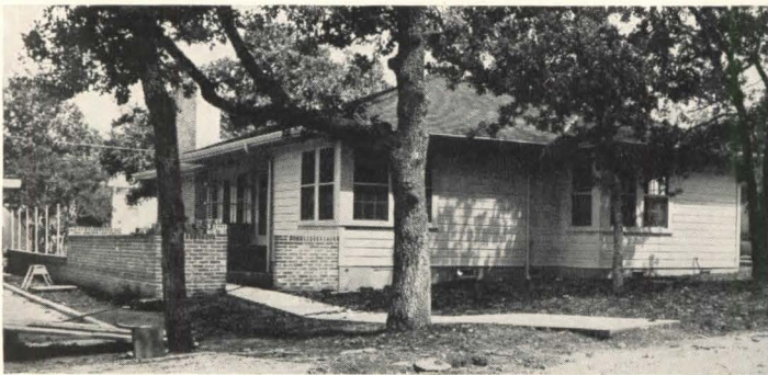
This frame house, similar in size and plan to the ceramic houses, was used as a comparison to demonstrate how much cooling could be stored in the heavy walls of ceramic tile and brick
