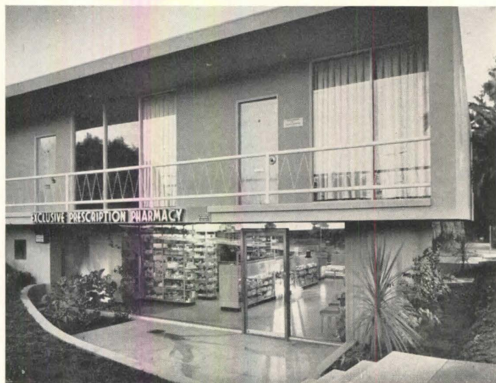
Above, left: one of the four units fully equipped for dental use. Above, right: main entrance to pharmacy. Below: rear of building; stairs lead to patio-lobby; rear entrance to pharmacy is at ground level at foot of stairs. Foundation was recessed to heighten effect of unbroken surface of end walls
