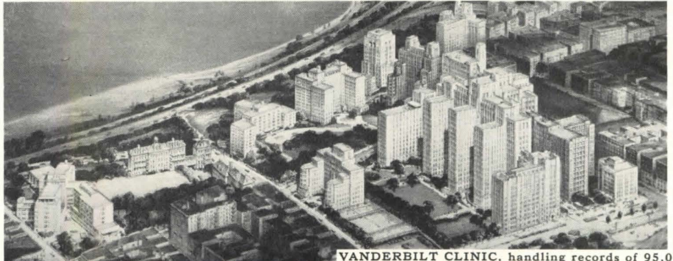
VANDERBILT CLINIC, handling records of 95,000 patients yearly, needed a fast, dependable system for transferring records from floor to floor, chose the VMP Conveyor.
