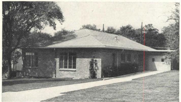
Another house being tested to obtain data on natural cooling of tropical houses is constructed of brick walls backed up by tile
