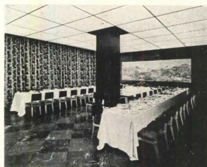
Plastic sheets used in luminous ceiling at Hotel Sheraton in Pittsburgh
