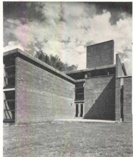
Ground-level entrance to teaching studios, rehearsal rooms, maintenance areas
