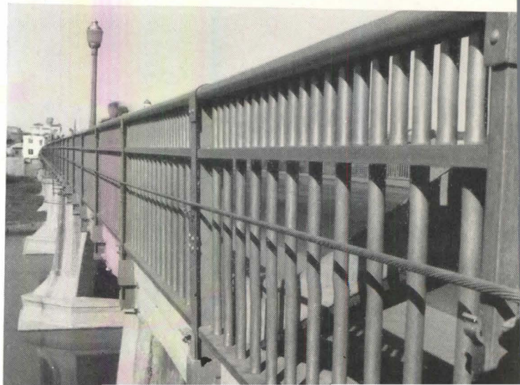
International Bridge, Laredo, Texas, has aluminum railings installed in 1935. In the event of floods, the entire railing can be quickly removed.
