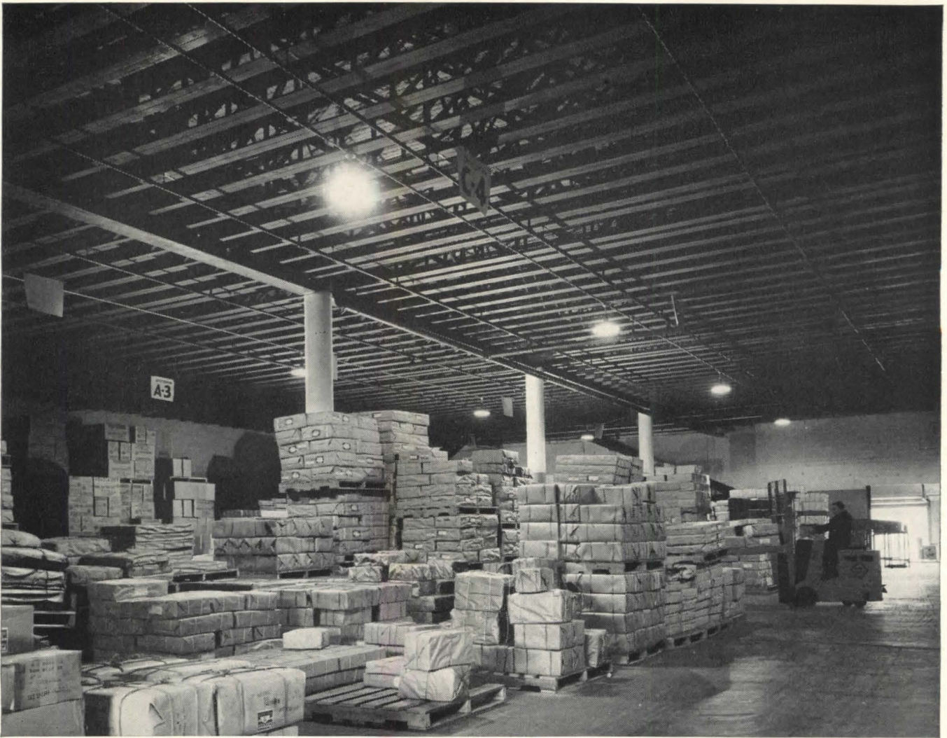
Bethlehem Longspan Joists provide greater usable floor space in H. J. Dowd Co., Inc. warehouse, Cambridge, Mass. Contractor: Earl Brown, Inc., Malden, Mass.; Architect: E. K. True, Concord, Mass.
