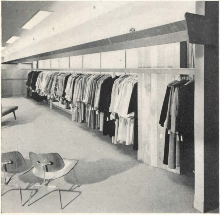
Above: air conditioning ducts are supported by patented steel struts and screened with perforated asbestos cement panels; panels are yellow, vents are bright red. Right: the architects designed dress and skirt racks and display cases
