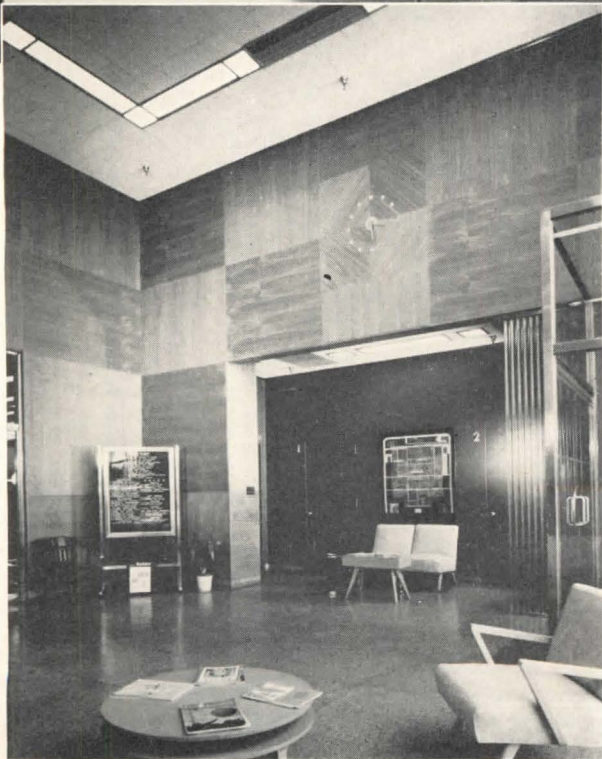
Main entrance lobby, above, is done with the same simplicity that characterizes the exterior. It opens into a products display room (center photo). Office areas and drafting rooms are kept just as open and flexible as the production areas
