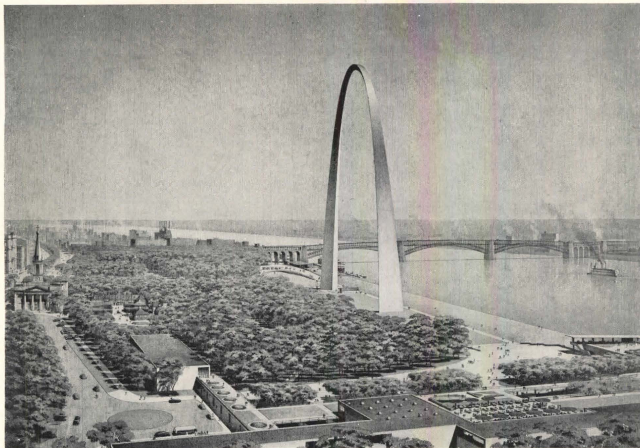
590-ft Jefferson Memorial Arch symbolizes the city of St. Louis as gateway to the West. Heavy stainless steel was chosen for the covering to insure durability and to prevent ripples which might make it look "tinny"
