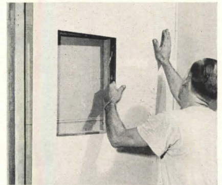
Moisture-proof plastic panels are used for wall board (above), reveals (below)
