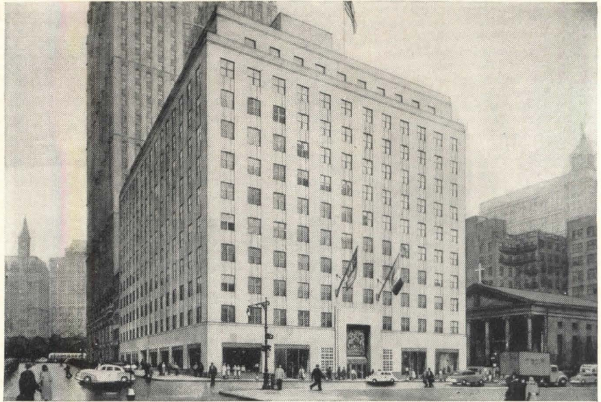
NEW DUN & BRADSTREET BUILDING in New York City has G-E Personal Weather Control Air Conditioning. Over 450 G-E room units circulate filtered, fresh air that is cool in summer, warm in winter. Architect: Reinhard, Hofmeister, & Walquist. Consulting engineer: Syska & Hennessy, Inc. General contractor: George A. Fuller Company. Air conditioning contractor: Kerby Saunders, Inc.
