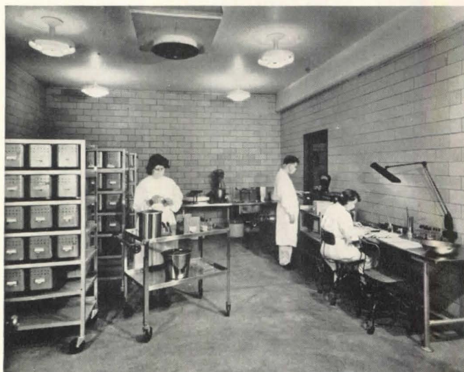
Above right: virus laboratory in the biological wing is completely isolated from rest of building, entered by air locks and on separate air conditioning system, maintaining negative pressure. Above left: mouse room, biological wing. Below: a more or less typical biochemistry laboratory
