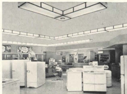
20% MORE LIGHT! Here is MODULE in an appliance store, delivering 70 footcandles. Using the same number of ordinary fixtures, only 58 footcandles would be obtained.
