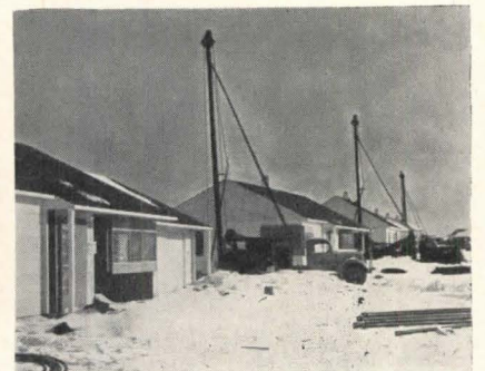
Plastic pipe is used to save cost in well installations for housing project
