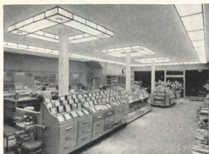
20% MORE LIGHT! In this modern drug store, MODULE attains a 96 footcandle output. An equivalent number of conventional fixtures would deliver only 80 footcandles.
