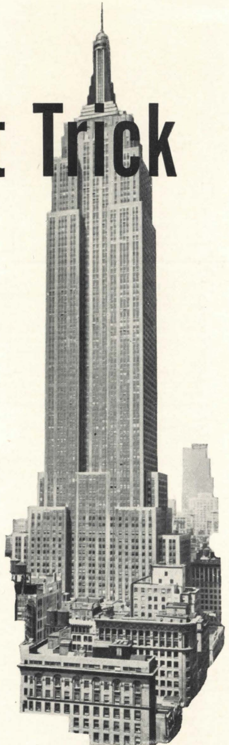
Consulting Engineer: Edward E. Ashley General Contractor: Starrett Brothers & Eken, Inc. Mechanical Contractor: Almirall & Co., Inc.
