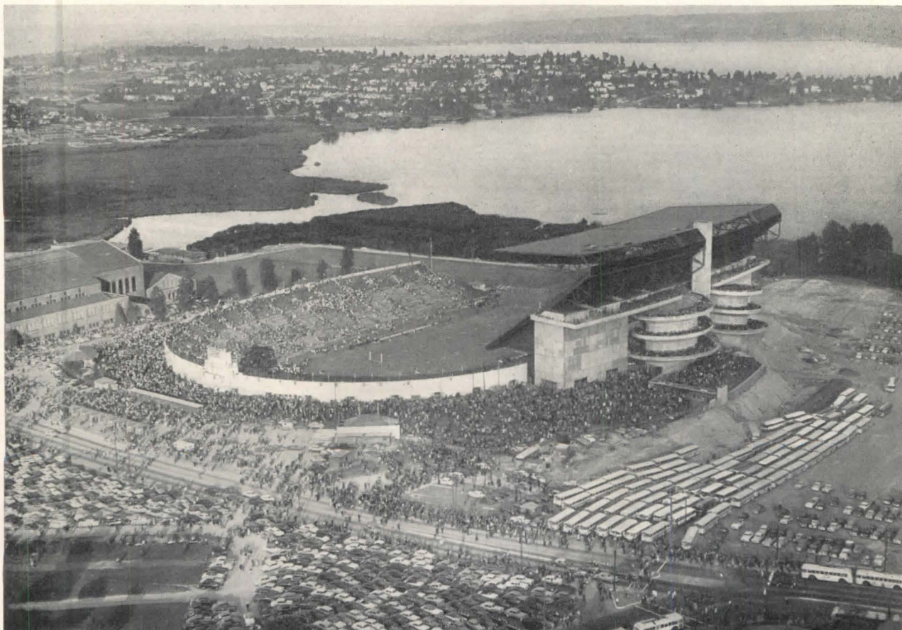
Below: concrete ramps as a means of circulation to the stadium addition were chosen because of the unidirectional traffic flow
